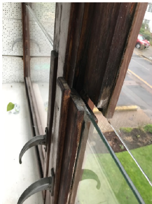
Casements either do not close or not able to be opened
