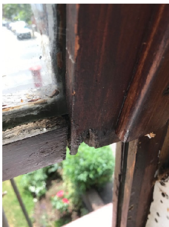
Casements either do not close or not able to be opened
