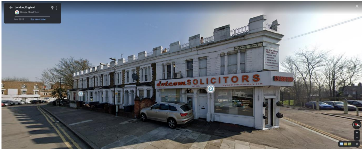
Fig. 2: Front elevation of Rawlinson Terrace shows the modern shop windows frontage at Ground Floor of no. 352 – 354.
