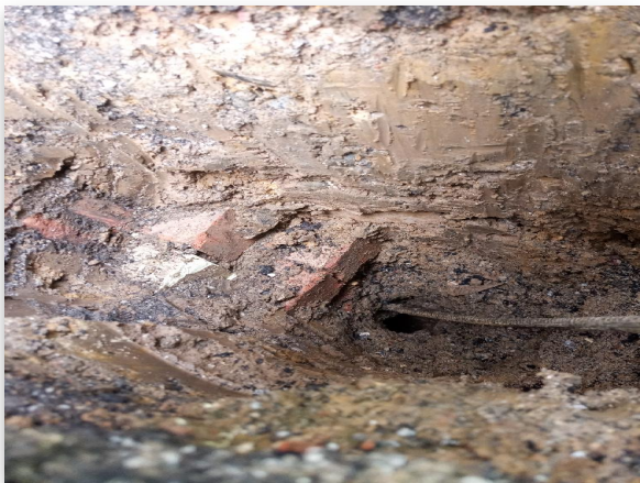
Fig 1.2: Trial Hole 1 Footing
