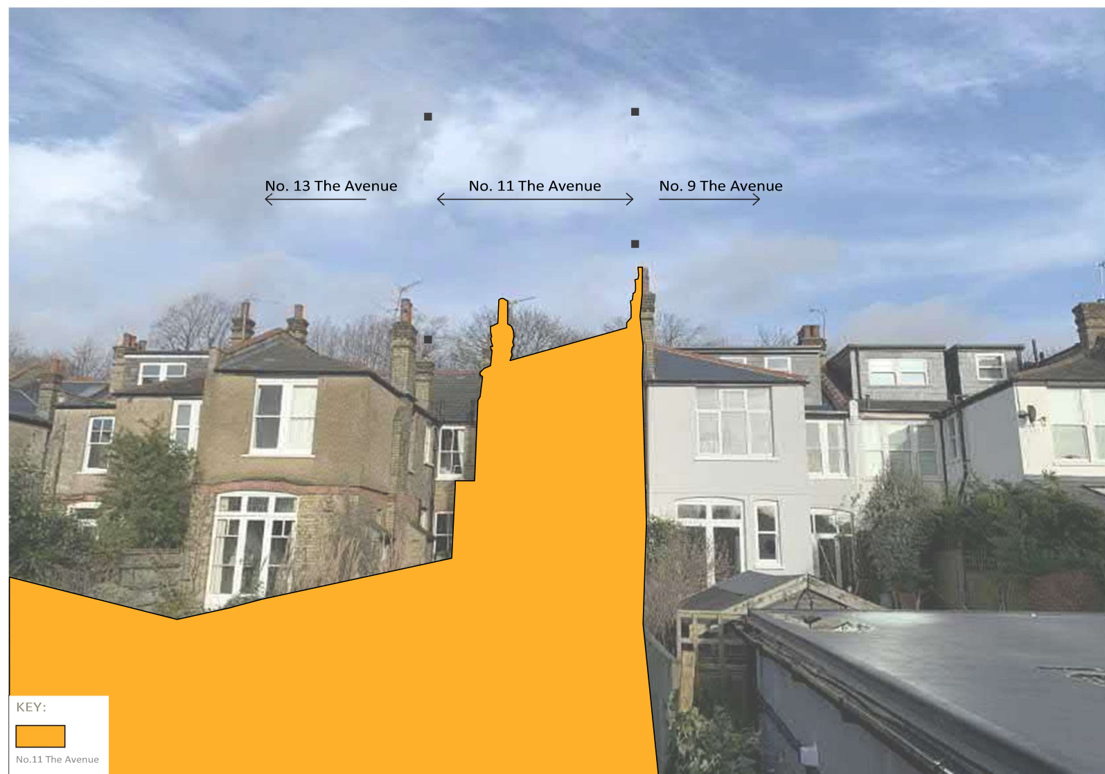
Image 10. View to the rear of the property
