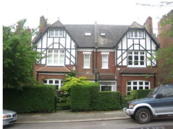
9-47: 10 pairs of semi-detached houses, early 1890's, built by the IPIC, half-timbered type (as Onslow Gardens)
