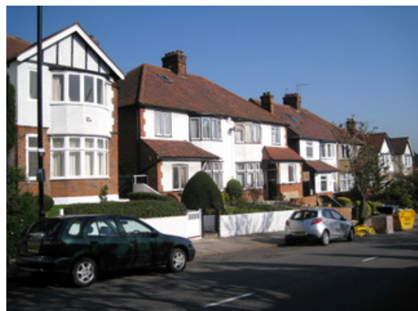
2-12: four pairs of semi-detached and two detached houses built in the 1920's, two-storey with bays on ground and first floors.
