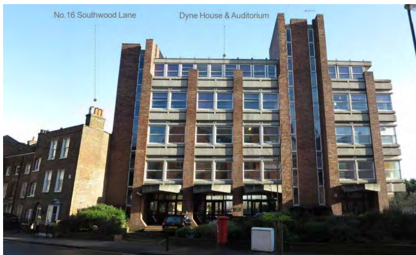
Figure 5: Existing Front Elevation Dyne House
