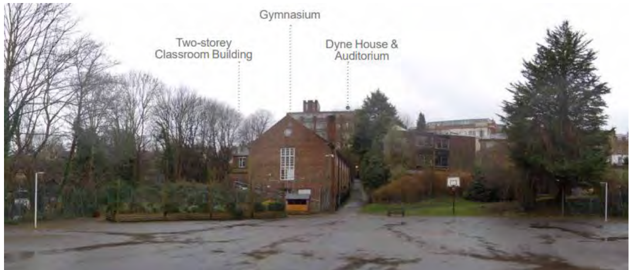
Photo of Rear Elevation
