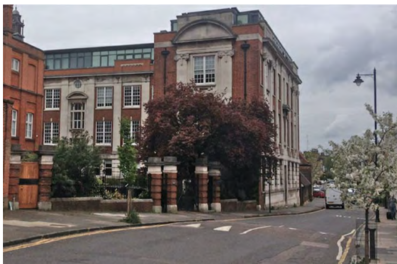
Figure 9: Existing Science Block
