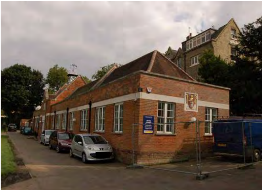
Figure 11: Existing Richards Music Centre
