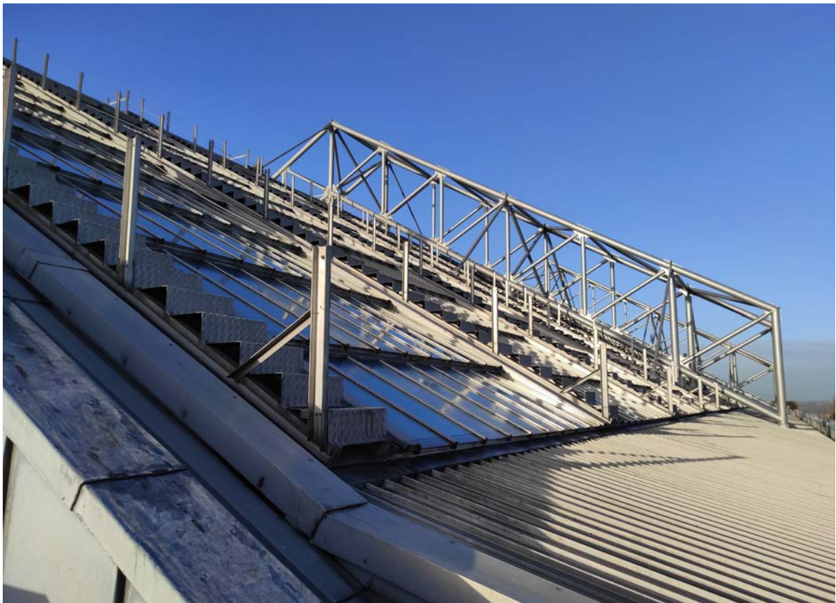
Figure 11: Existing space frame roof structure and maintenance roof access stairs.
