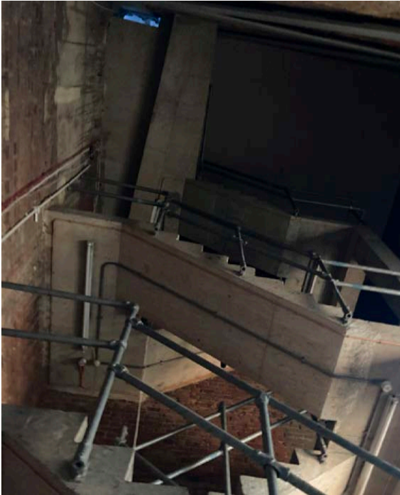
Figure 6: Existing non-original concrete stair and scaffold balustrade access to roof.
