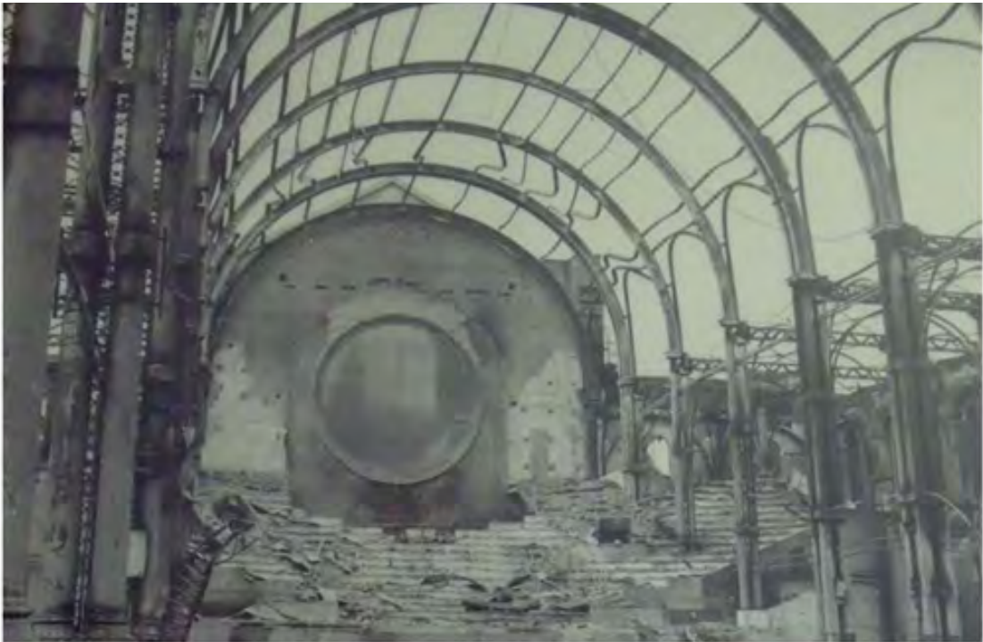
The Great Hall after the 1980 fire - View towards the North
