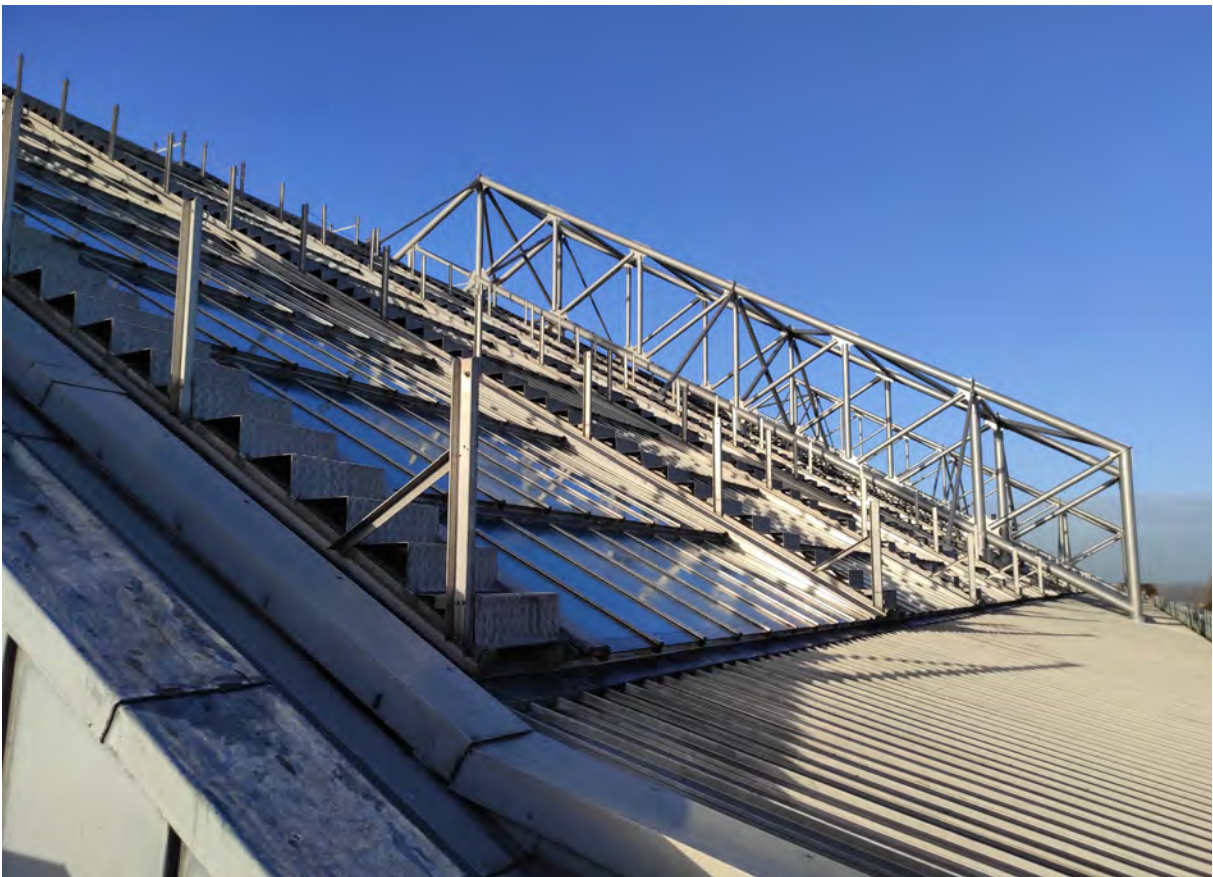
Figure 11: Existing space frame roof structure and maintenance roof access stairs.
