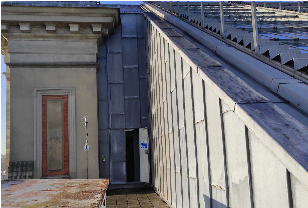
Figure 10: Existing area of roof accessed from the top of the internal concrete stair
