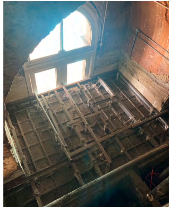
Figure 9: Non-original ceiling to East lobby
