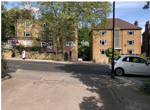
Apartment buildings opposite Alford House on Stanhope Road
