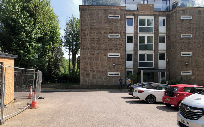
Existing car park and its relationship with 1-16 Alford House
