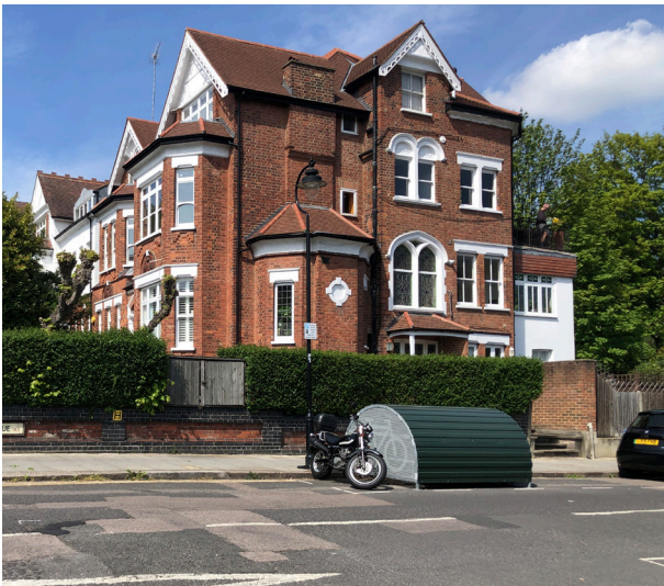
Existing townhouses on Stanhope Road
