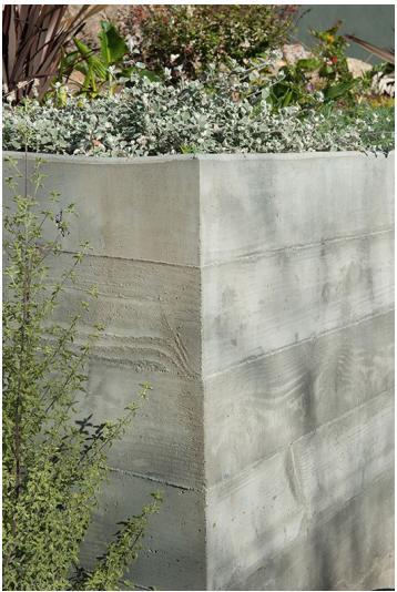
Proposed wood board shuttered concrete details
