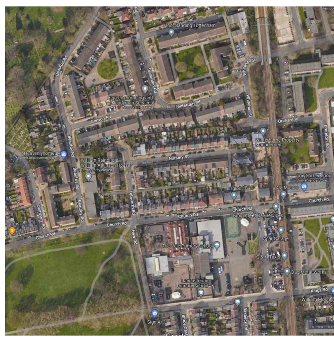
25 AERIAL PHOTOGRAPH SCALE N/A
