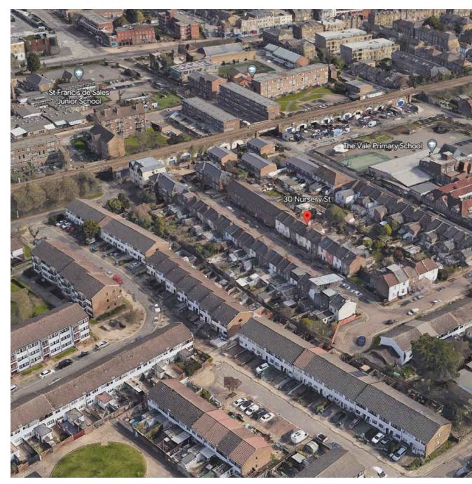
29 AERIAL PHOTOGRAPH SCALE N/A
