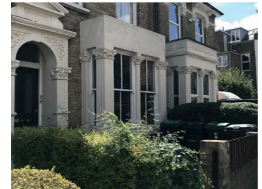
Whilst many of the traditional features are retained, many of the timber sash window have been replaced with poor quality UPVC window frames
