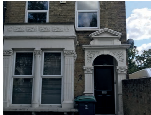
Whilst many of the traditional features are retained, many of the timber sash window have been replaced with poor quality UPVC window frames
