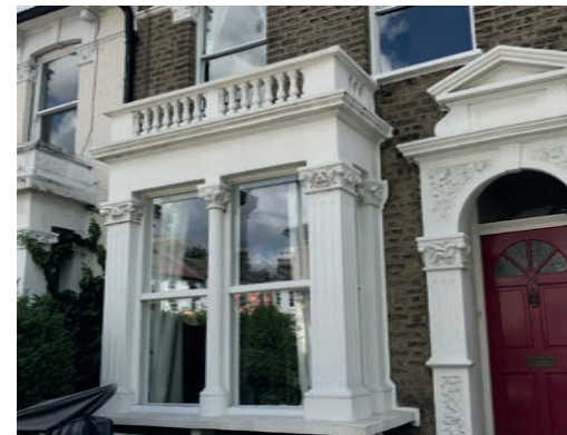
Whilst many of the traditional features are retained, many of the timber sash window have been replaced with poor quality UPVC window frames
