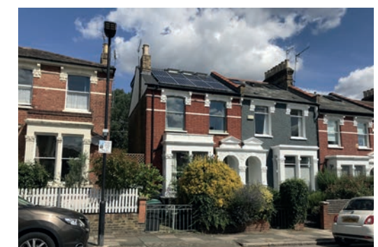
Whilst many of the traditional features are retained, many of the timber sash window have been replaced with poor quality UPVC window frames
