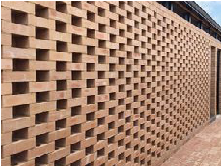
Perforated brick wall to northern boundary
