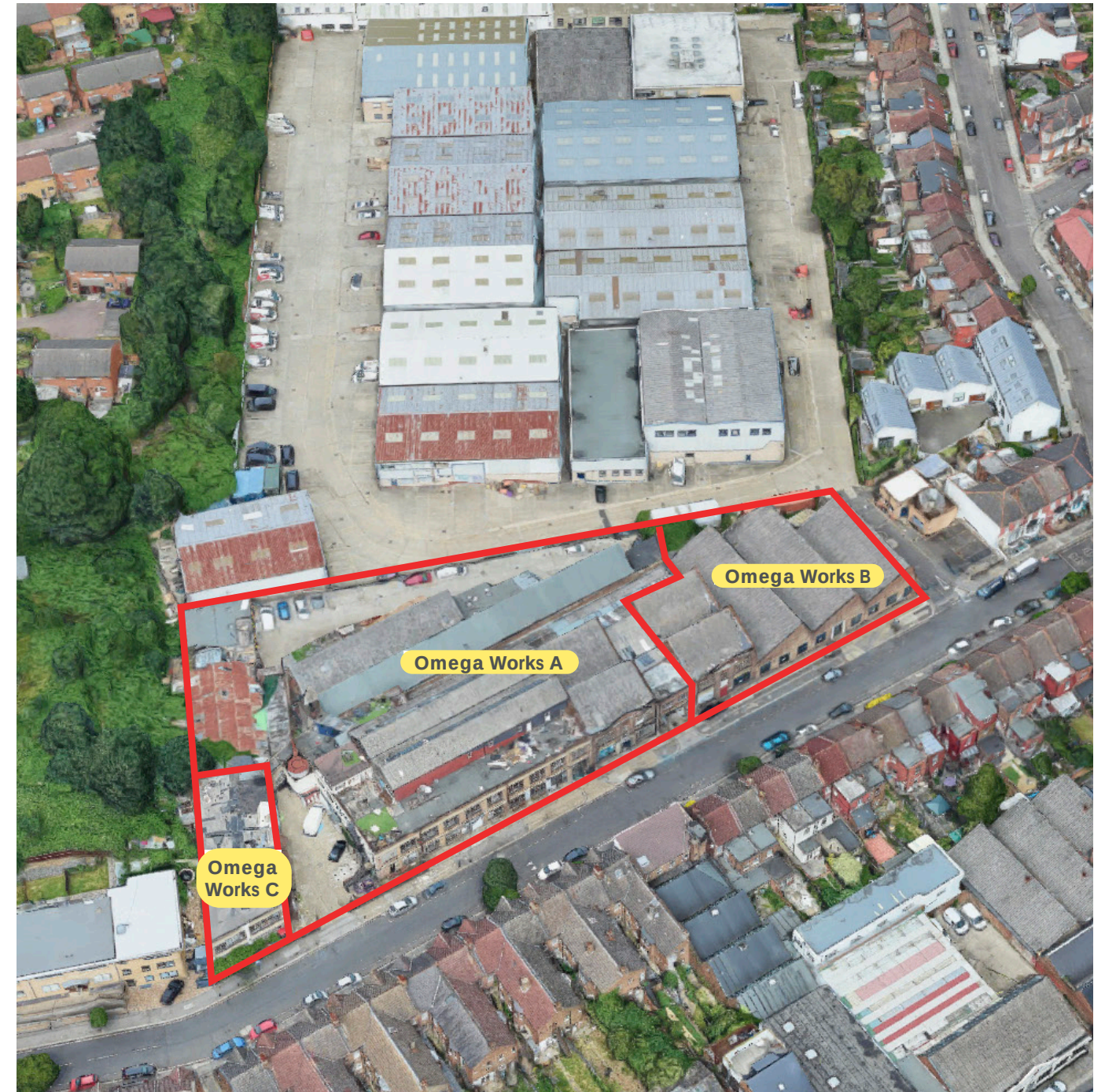
Aerial view of site illustrating the relationship between Omega A, B, C and respective red lines
