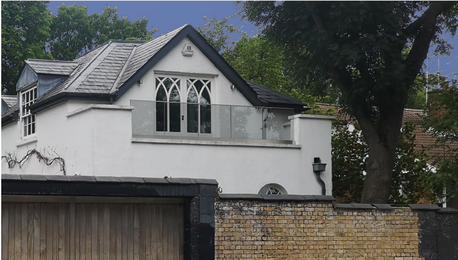
Existing Glass Railing
