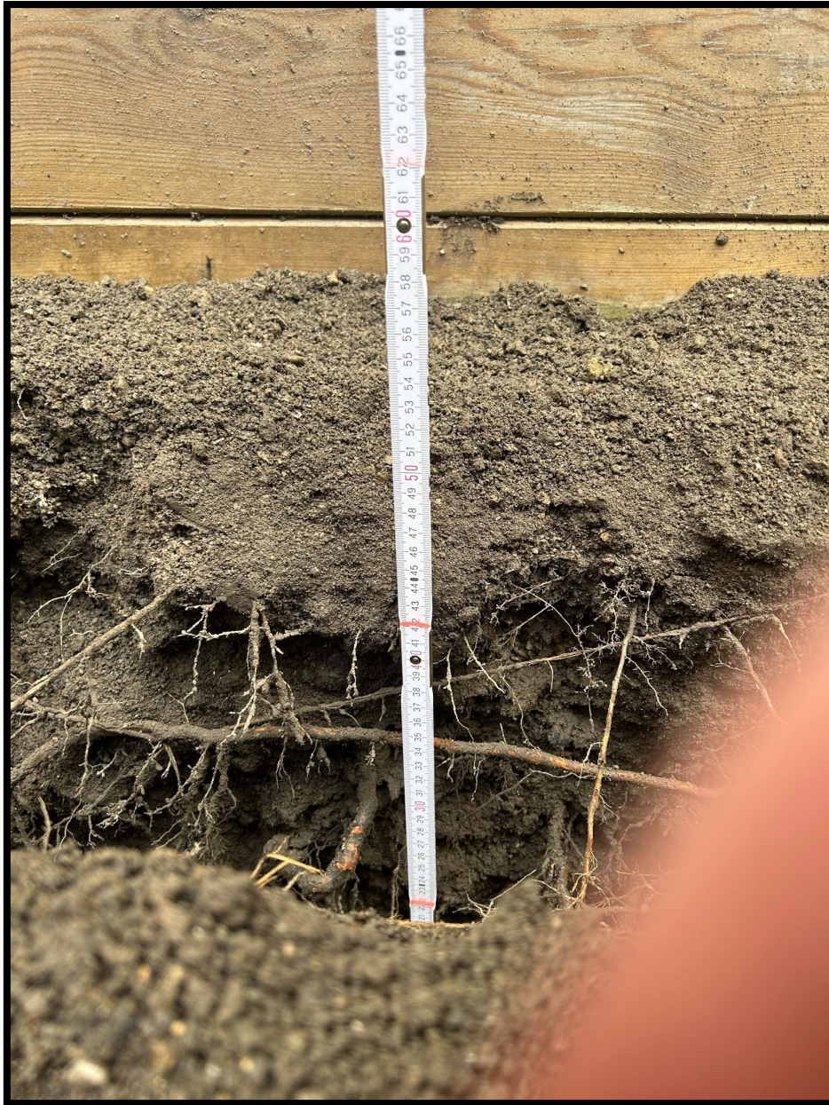
Figure 3 – Average depth of the excavation up to 600mm
