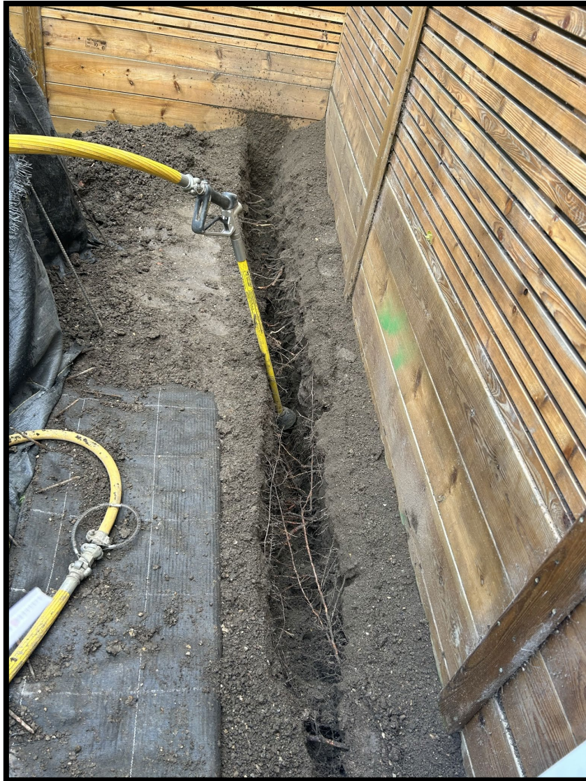
Figure 2 – Completed air spade trial excavation to a depth of 600mm.
