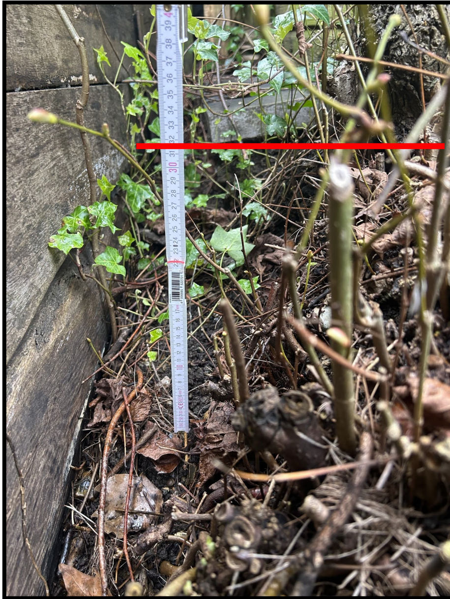
Figure 7 – Measurement of the stem location up the soil embankment, offsite. Stems are situated approximately 300mm up the slope, as noted with the red line.
