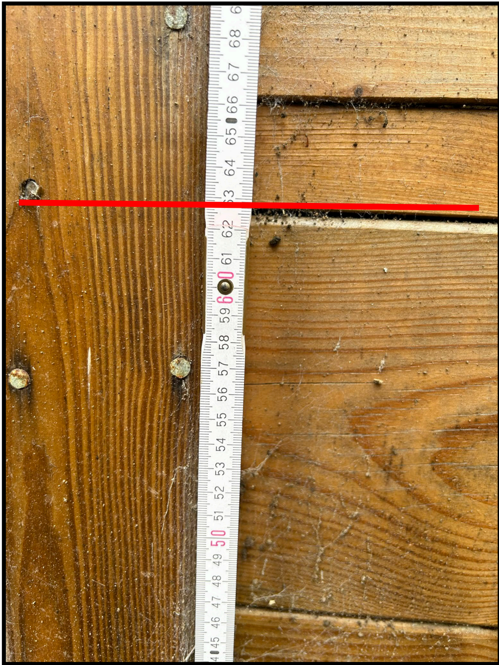
Figure 6 – Measurement of the level difference from within the Site – the red line denotes the approximate ground level on the other side of the fence
