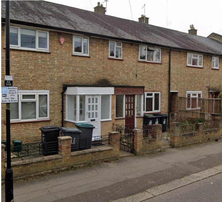
PICTURE: 1 Sample of existing porches at Farrant Avenue.
