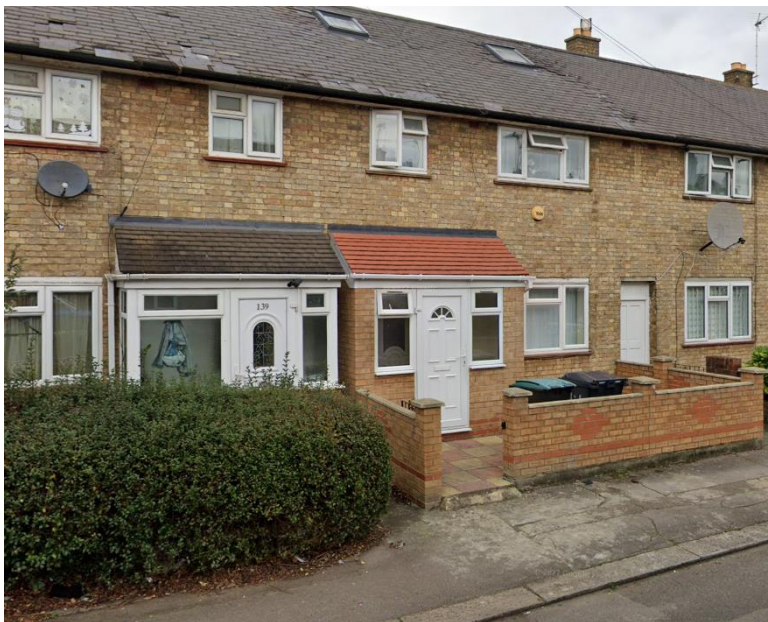
Picture: 2 Sample Of Existing Porches At Farrant Avenue.
