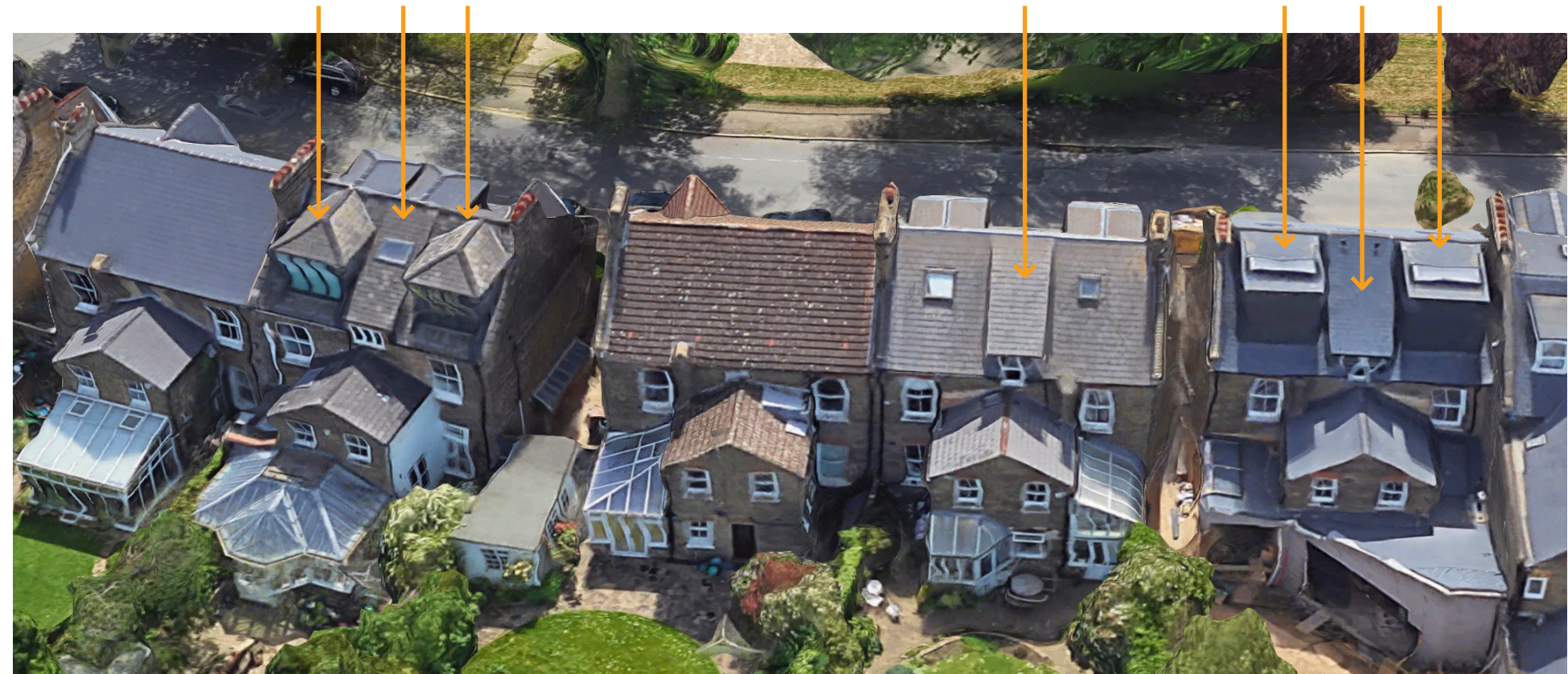
Rear of 59 - 67 Mount View Road showing rear dormers over the stairs and to the bedrooms in the converted loft space.
