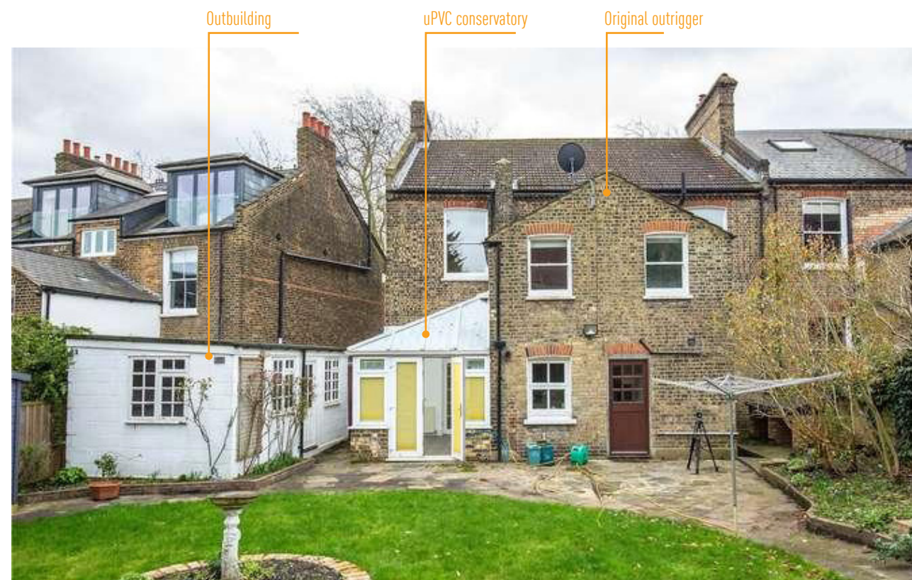
Rear of 63 Mount View Road showing the original outrigger in the centre, the uPVC conservatory to the side of it, and the outbuilding alongside the boundary with no. 65.
