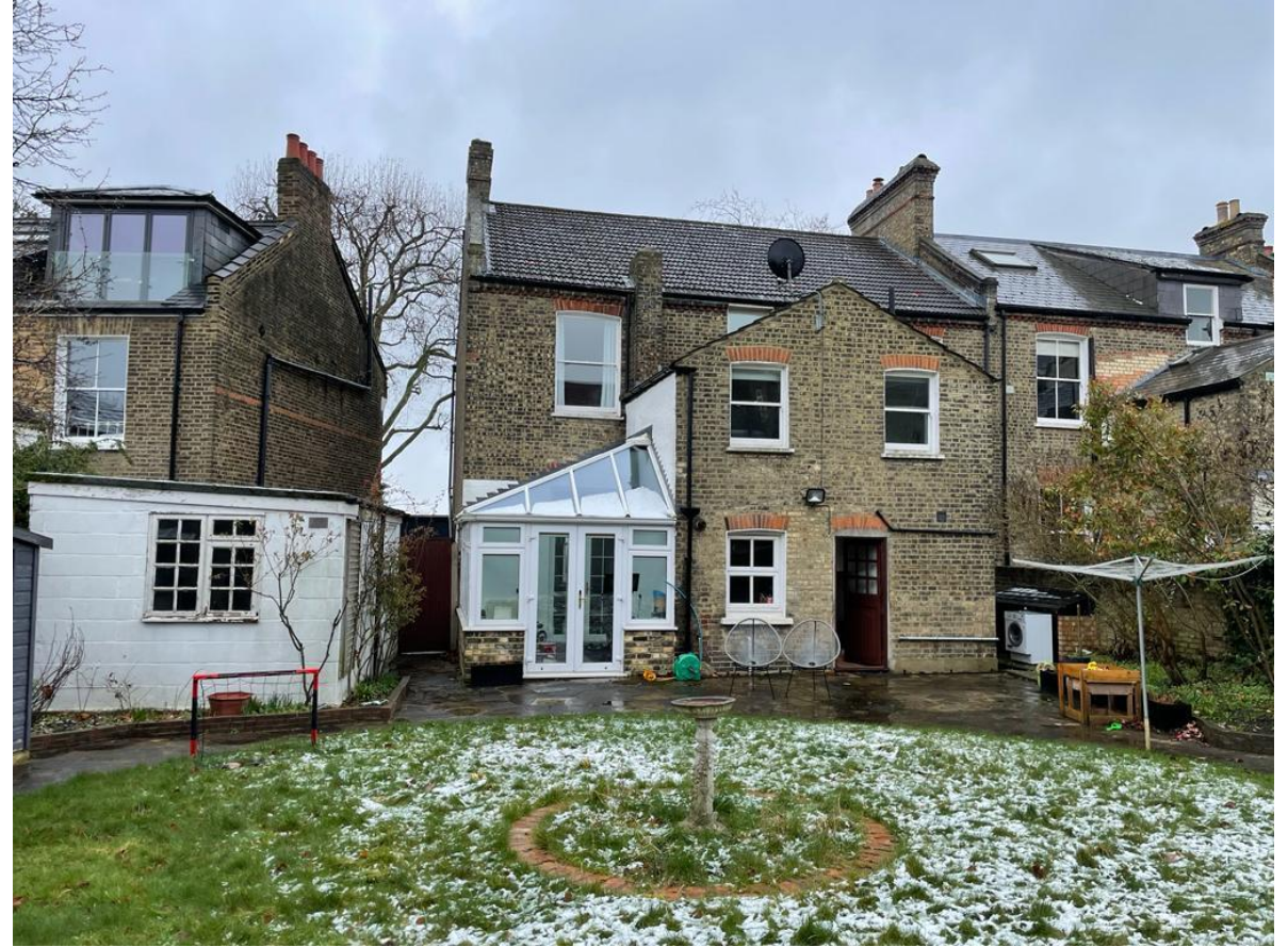
Photograph 8 – View of the rear of the property.
