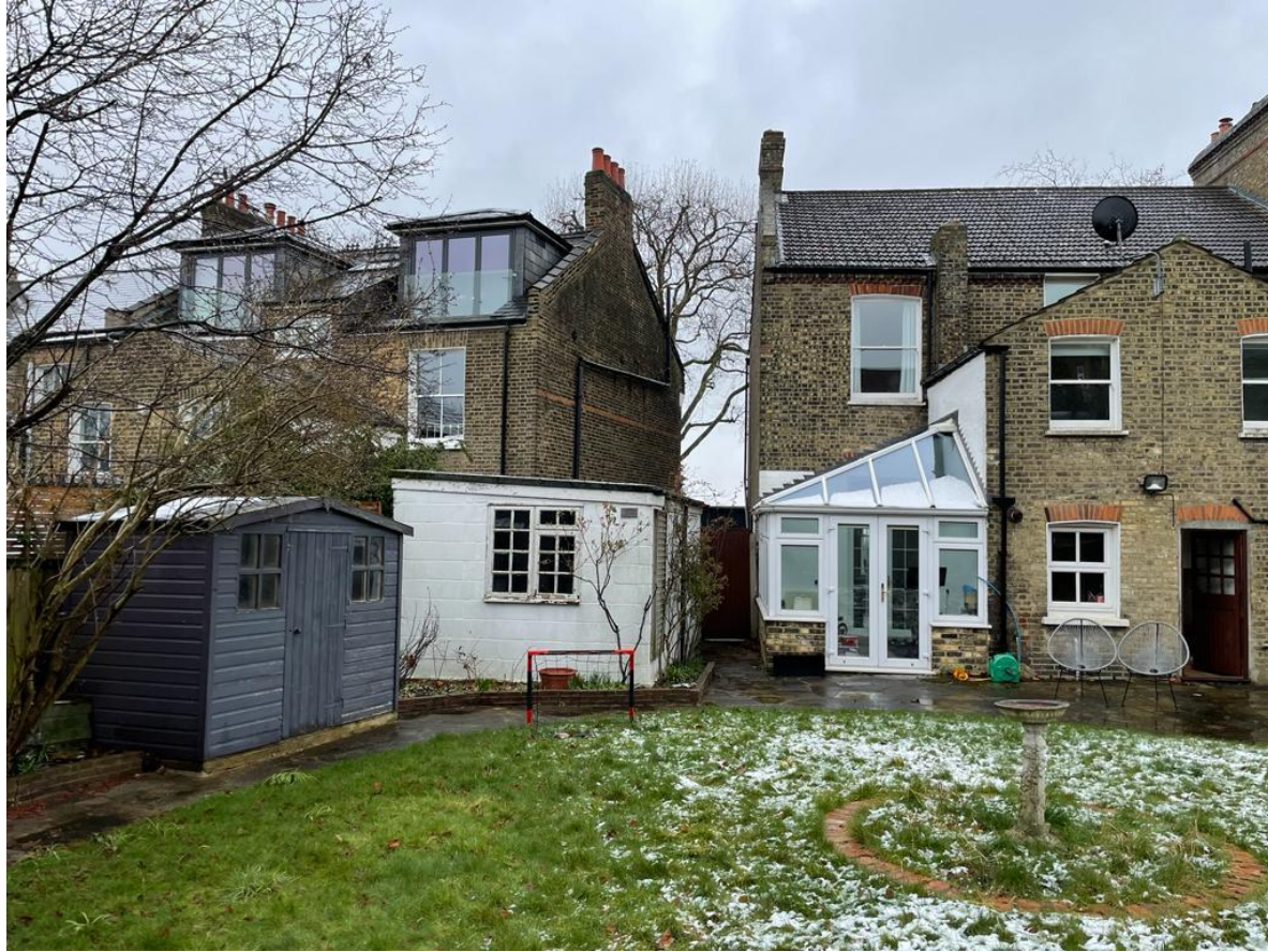
Photograph 9 – View of the shed and outbuilding at the rear of the property.
