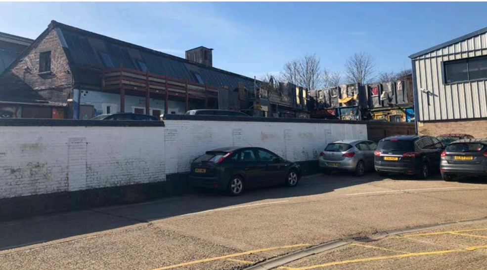
Photo of the existing rear boundary of Omega Works A, there is a large change in level as can be seen by the parked cars
