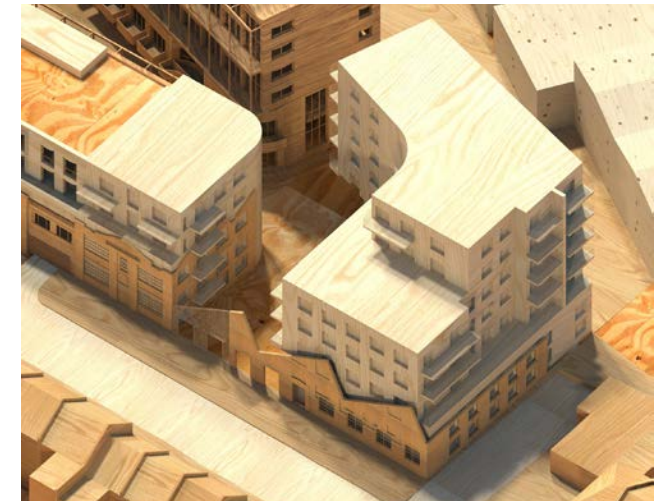
08. Balconies, Railings & Gates
