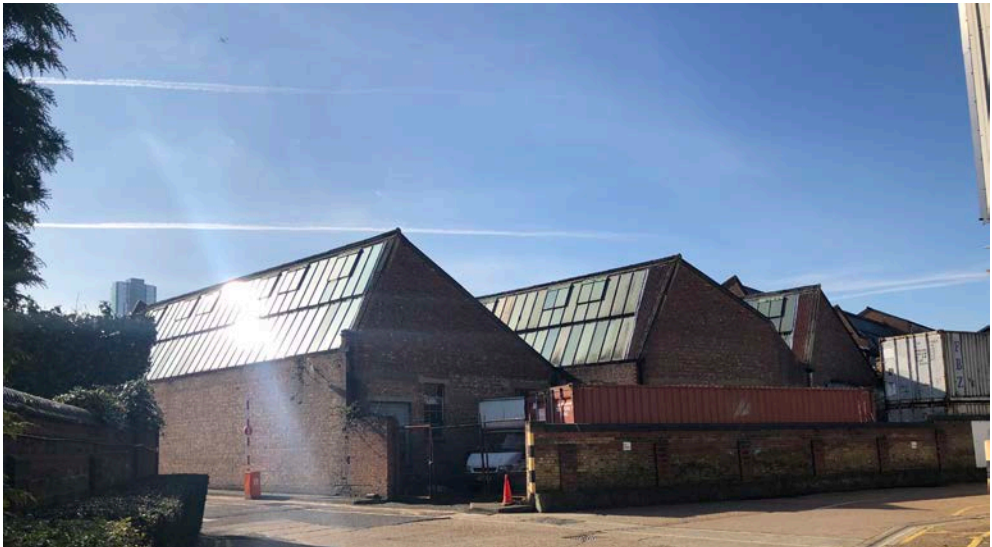
Photo of the existing rear boundary of Omega Works B there is a minimal change in level
