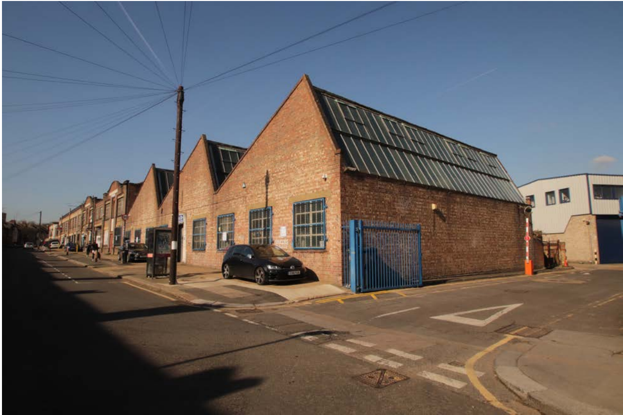
Omega Works viewed from Hermitage Lane
