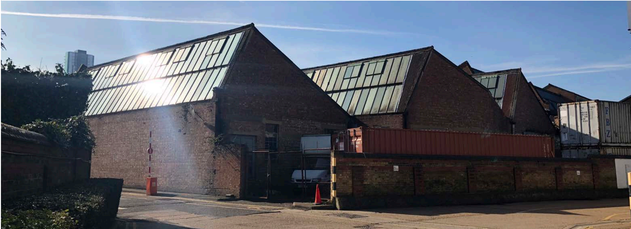
View from Crusader estate looking towards the site, there are no street trees affected by the works. As small area of Elder and Buddleia scrub will be removed to facilitate the works
