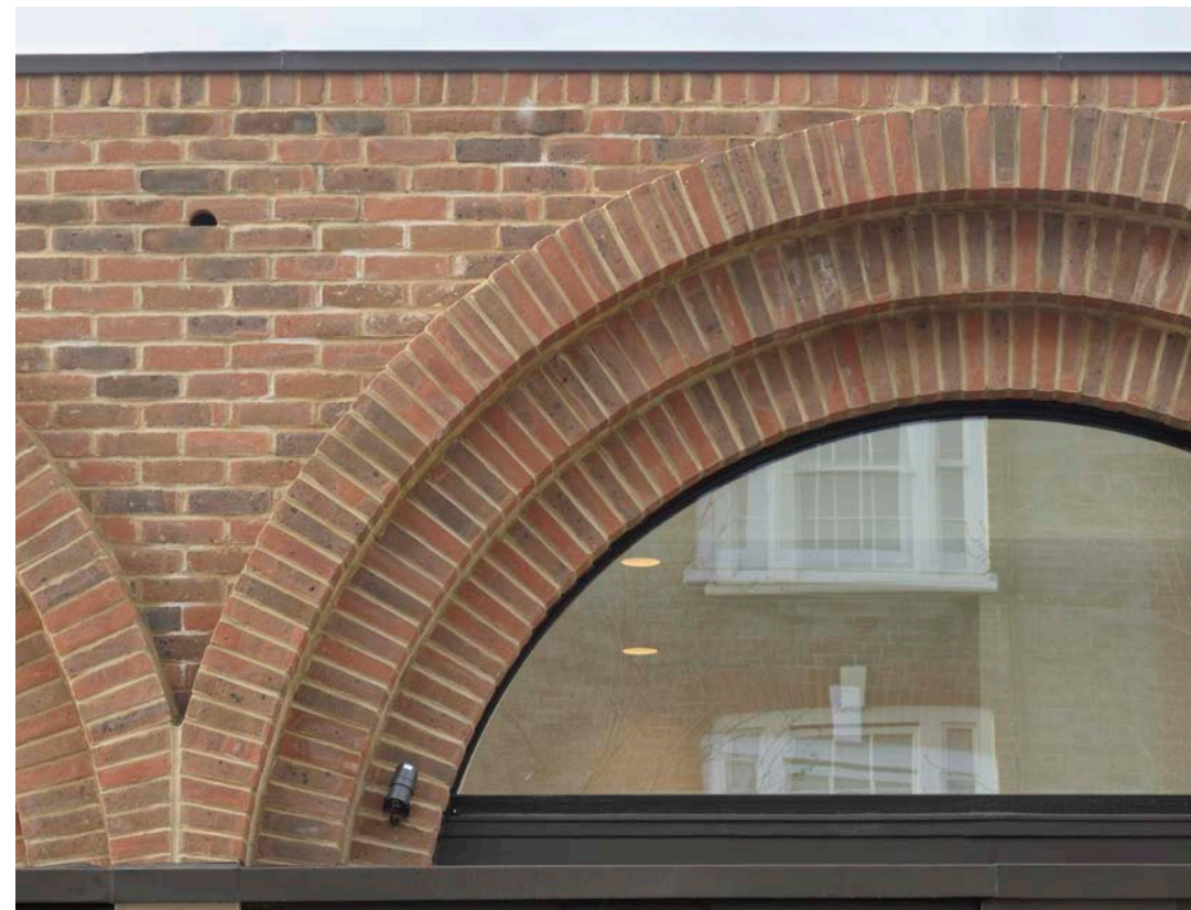
An installed example on a recent project by DHaus
