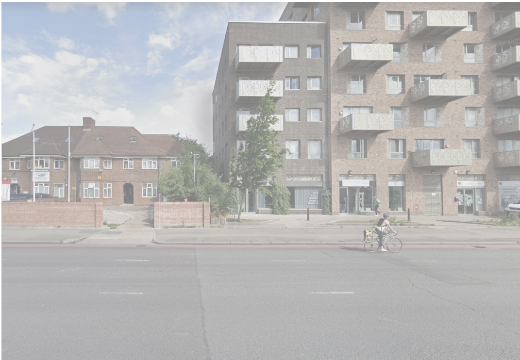
A 4m separation distance is visible between 307 and 309 Seven Sisters Road, the larger scheme recently approved by the Council
