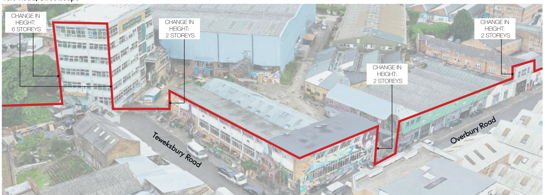
Tewksbury Road & Overbury Road, Streetscape
