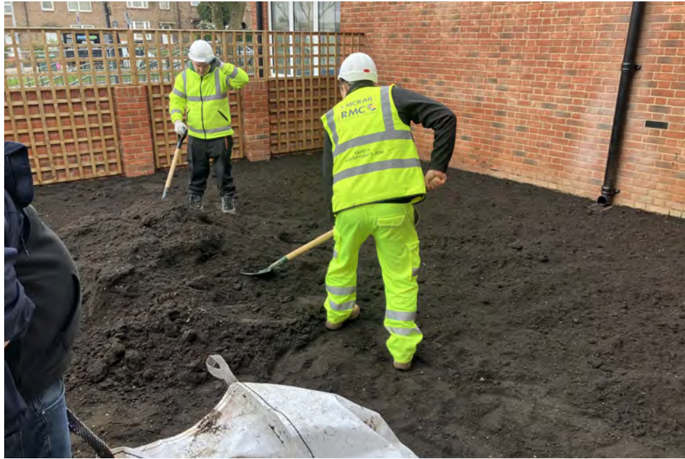
Topsoil Placement—H3 West 21/03/23
