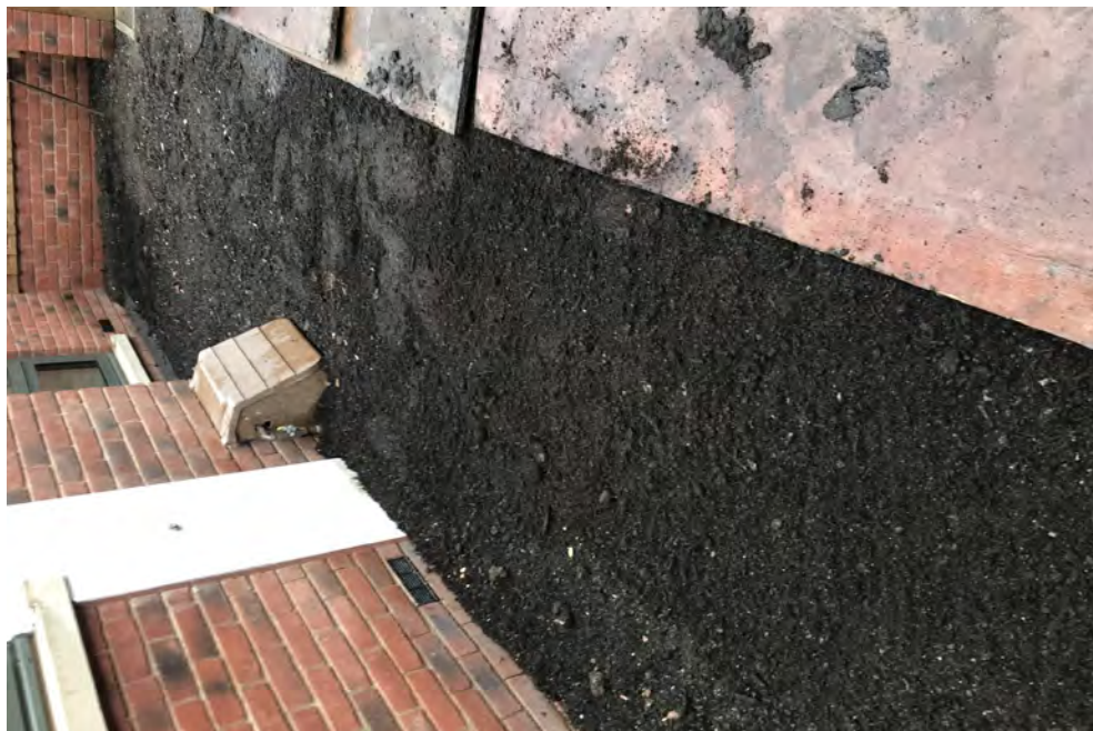
Vicarage East Small Topsoil Placed
