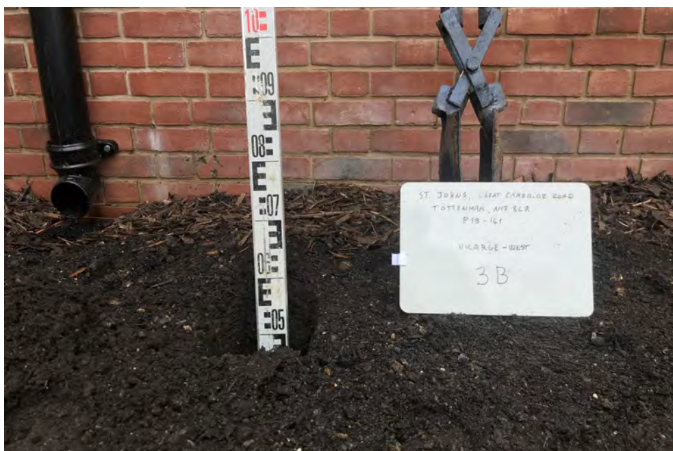
Topsoil Validation—Vicarage West Grid B3
