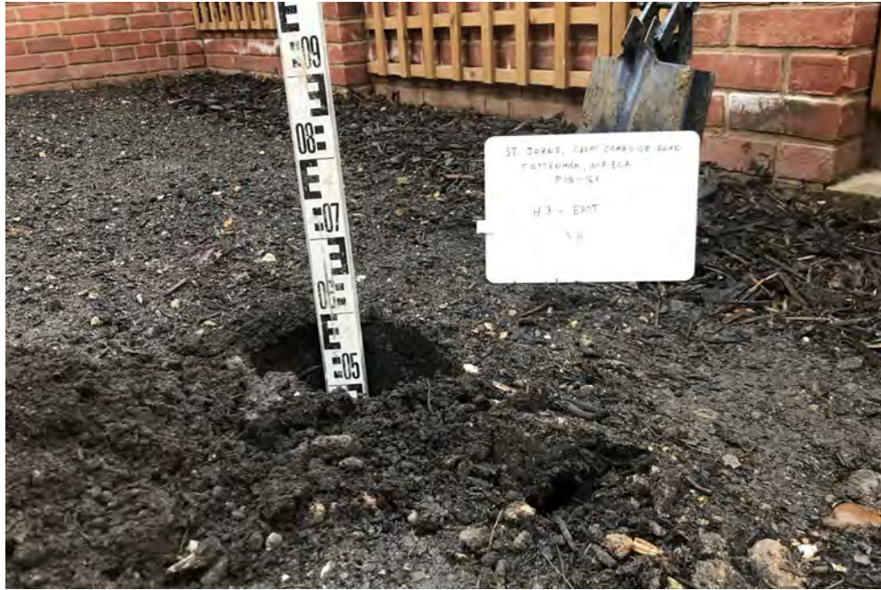
Topsoil Validation—H3 East Grid A3
