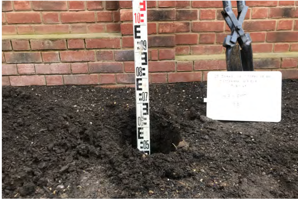
Topsoil Validation—H3 East Grid B2
