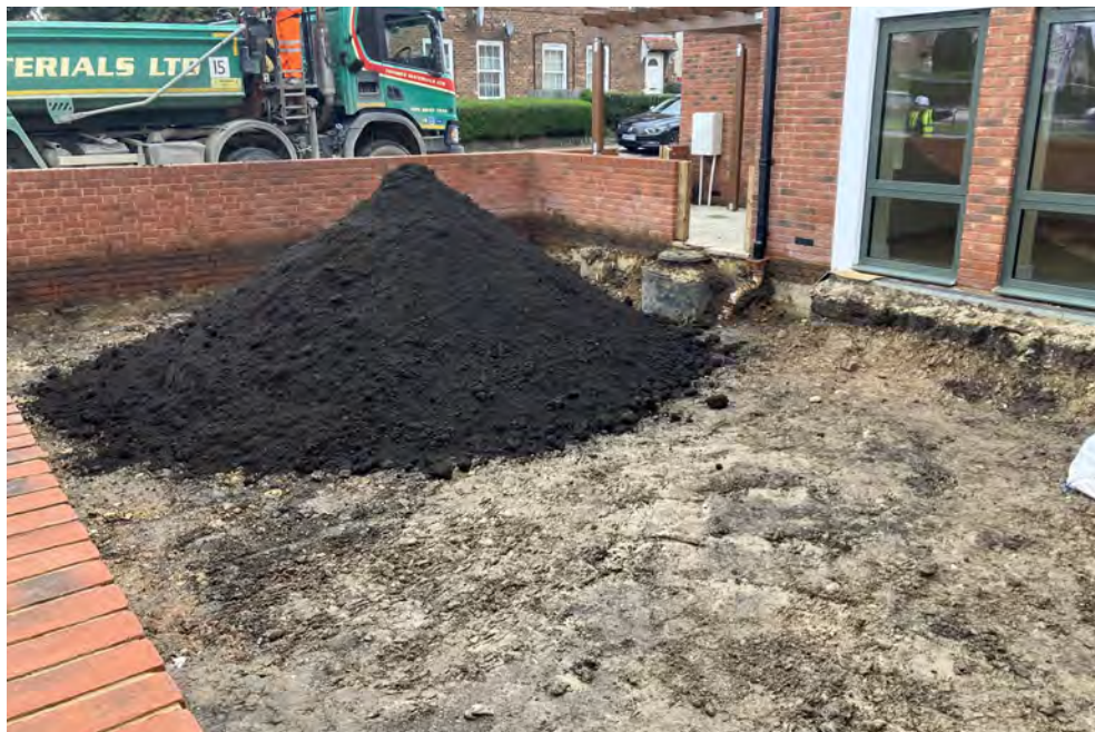
Topsoil Placement—Vicarage West 21/03/23
