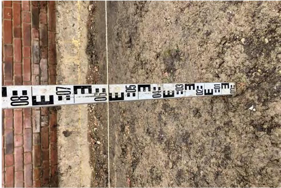
Formation Depth Check—Plot Vicarage West Grid B3
