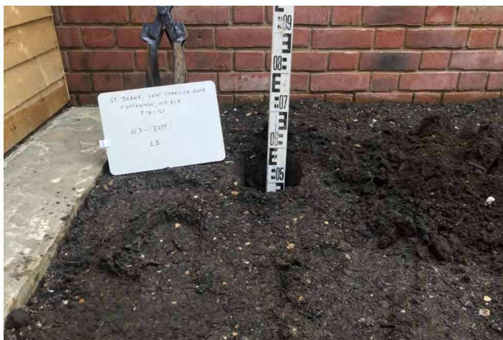
Topsoil Validation—H3 East Grid B1
