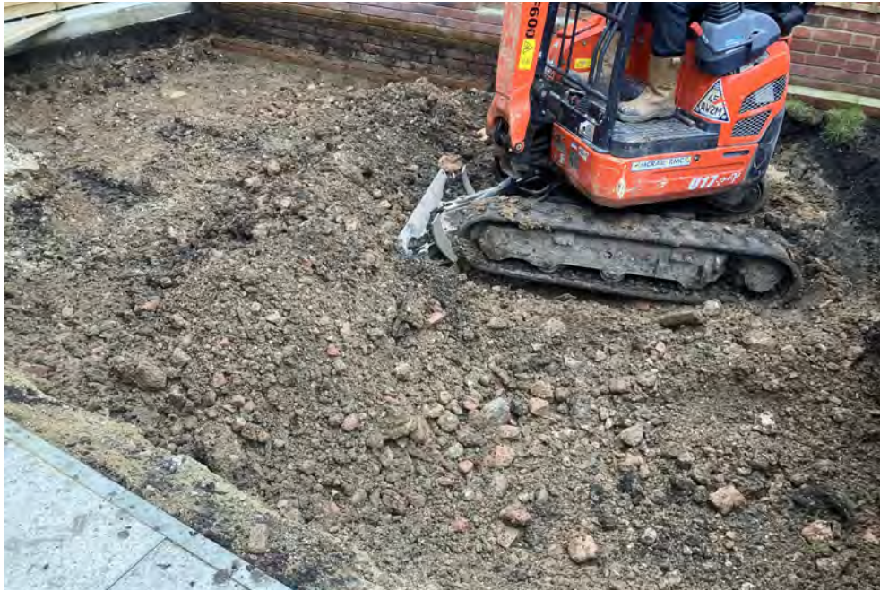
Plot H3 East in process of stripping to formation level
