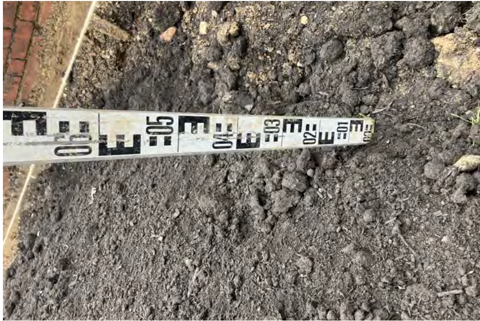
Formation Depth Check—Plot Vicarage West Grid B1
