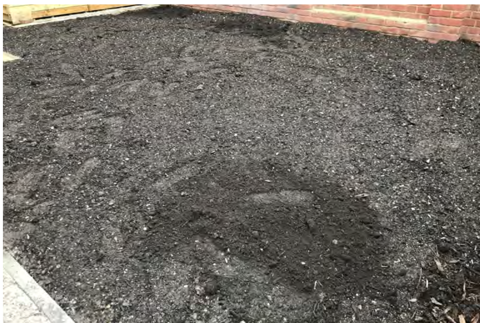
H3 East Topsoil Placed
