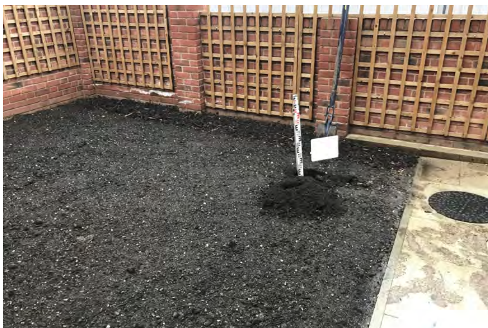
Topsoil Validation—H3 East Grid A3
