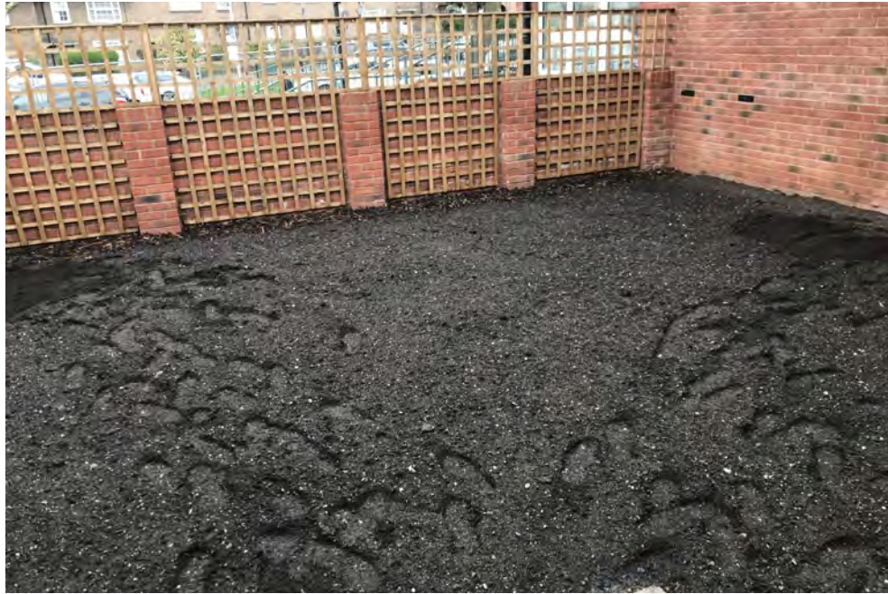
H3 West Topsoil Placed
