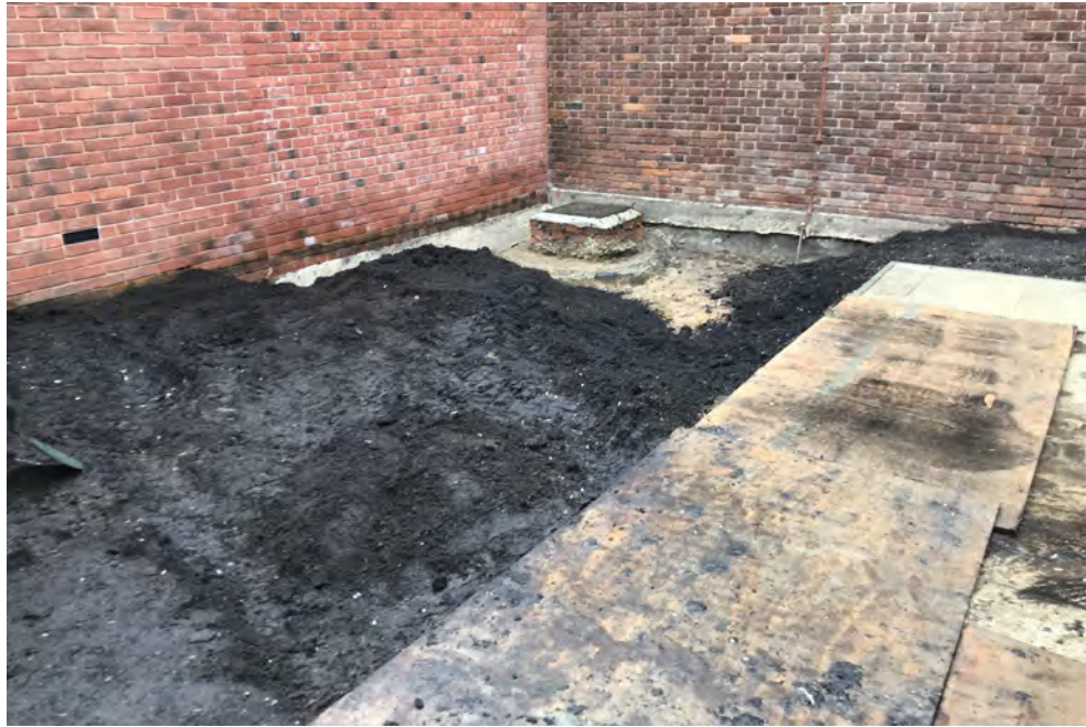
Vicarage East Large Topsoil Placed
