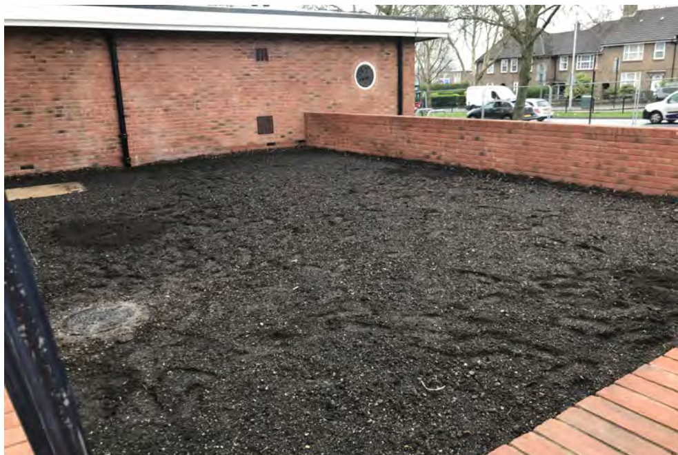
Vicarage West Topsoil Placed
