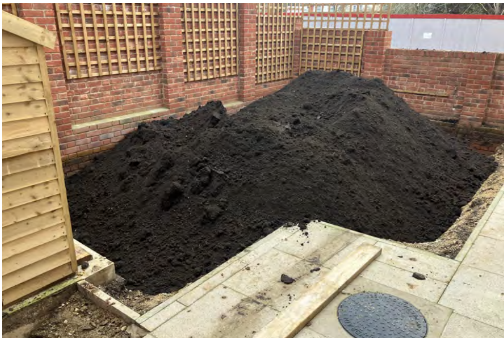
Topsoil Placement—H3 East 21/03/23
