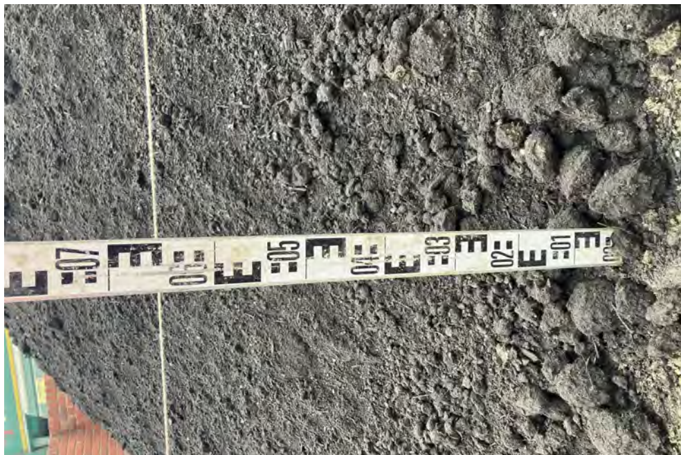
Formation Depth Check—Plot Vicarage West Grid B2
