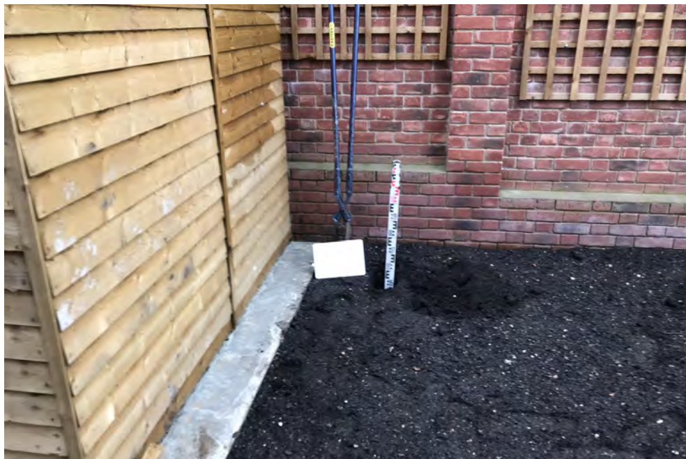
Topsoil Validation—H3 East Grid B1
