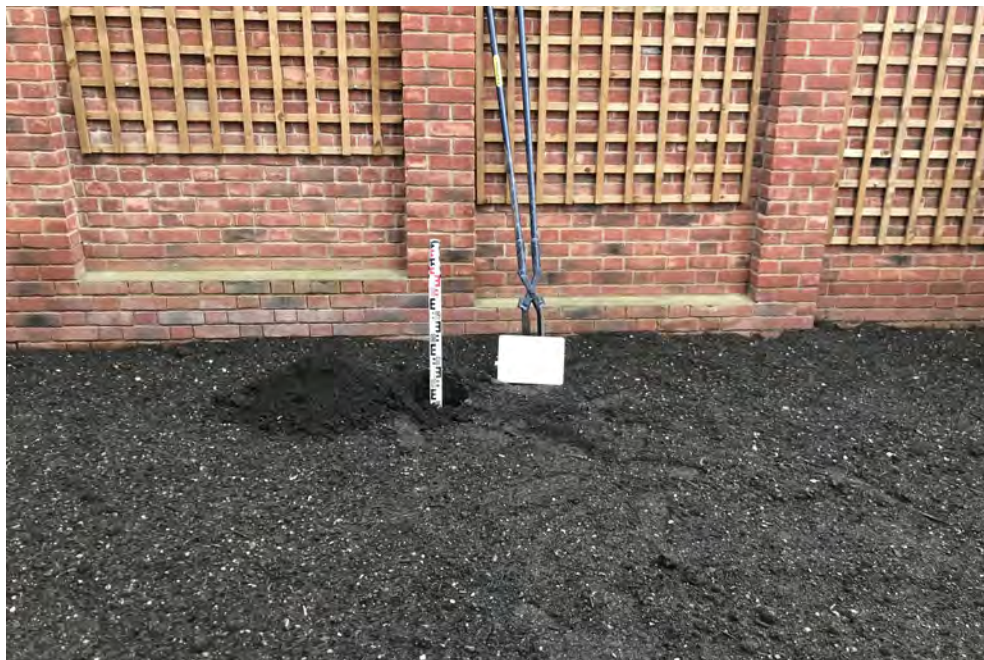
Topsoil Validation—H3 East Grid B2
