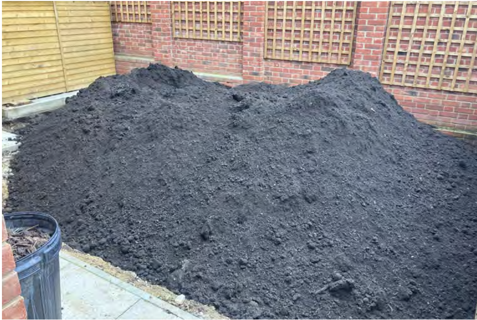
Topsoil Placement—H3 East 21/03/23
