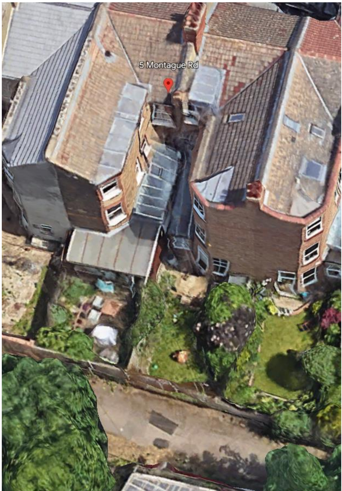
Aerial view of existing extensions to the rear of 5 Montague Road, N8 9PJ
