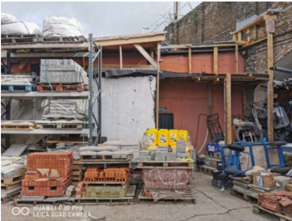
View to the left hand side of dilapidated building to show extent of current outside storage
