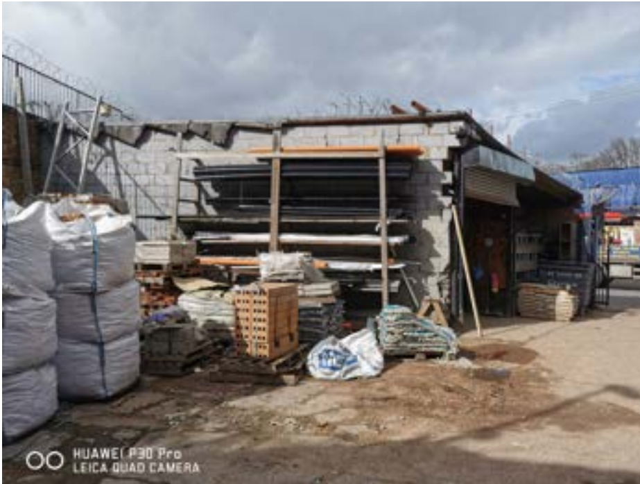
View to the left hand side of dilapidated building to show extent of disrepair
