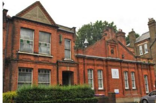
No 65, former Post office,, Southwood Lane
