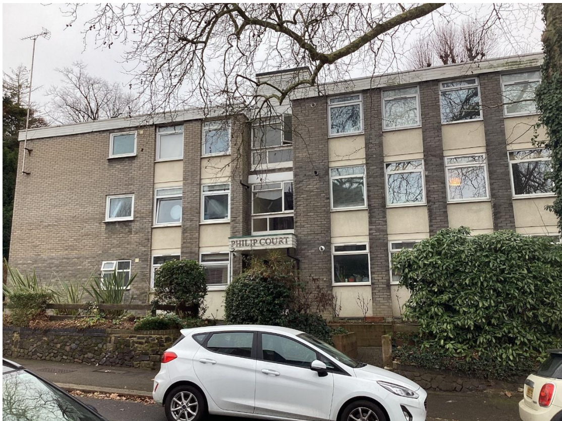
Figure 2 Philip Court (north east elevation).
