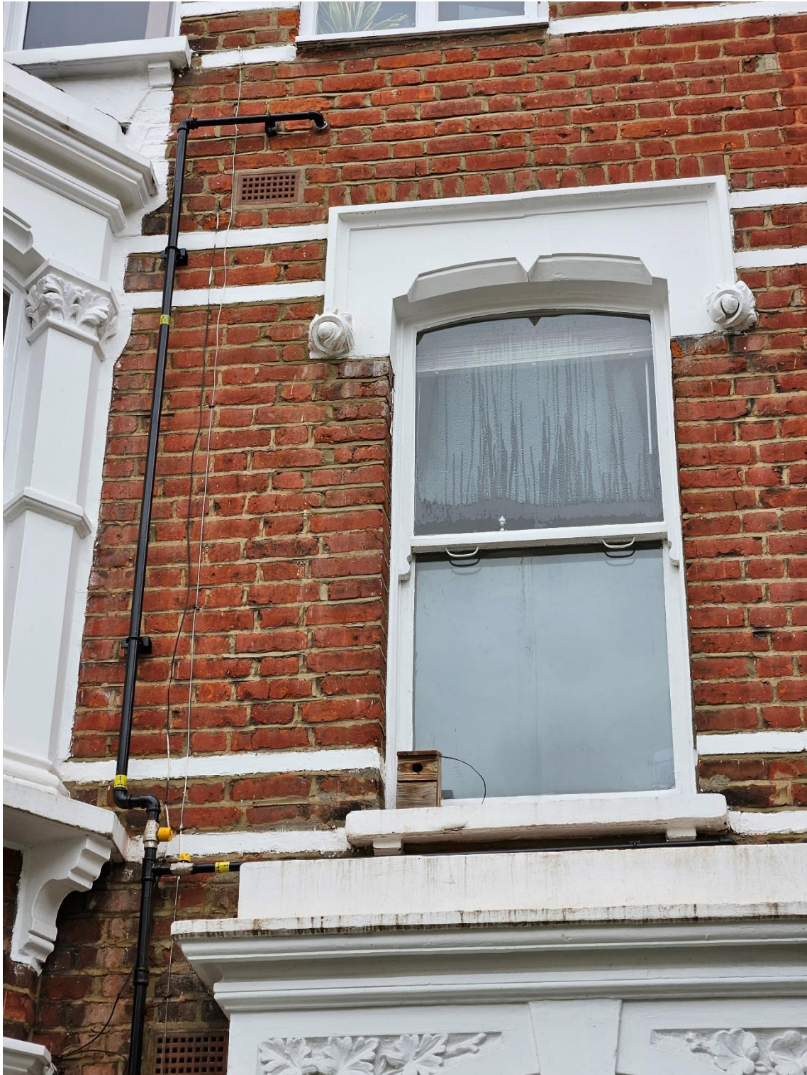
Figure 2 The installed gas riser to the first floor.
