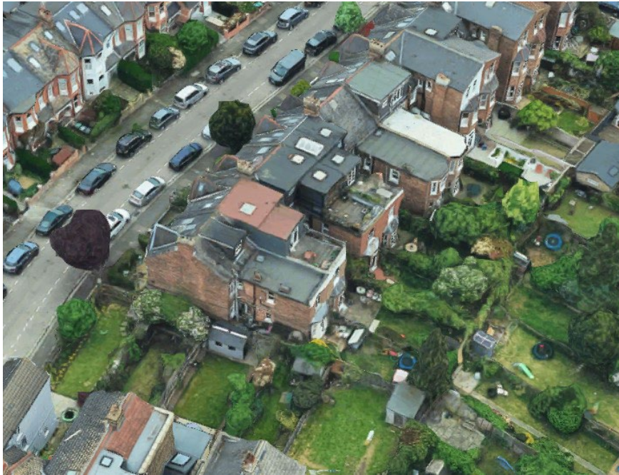
Photo 02 – Google 3D view with No 68B in the foreground and the roof extensions of Nos 66, 64 & 62 clearly seen
