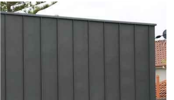
standing seam rainscreen cladding
