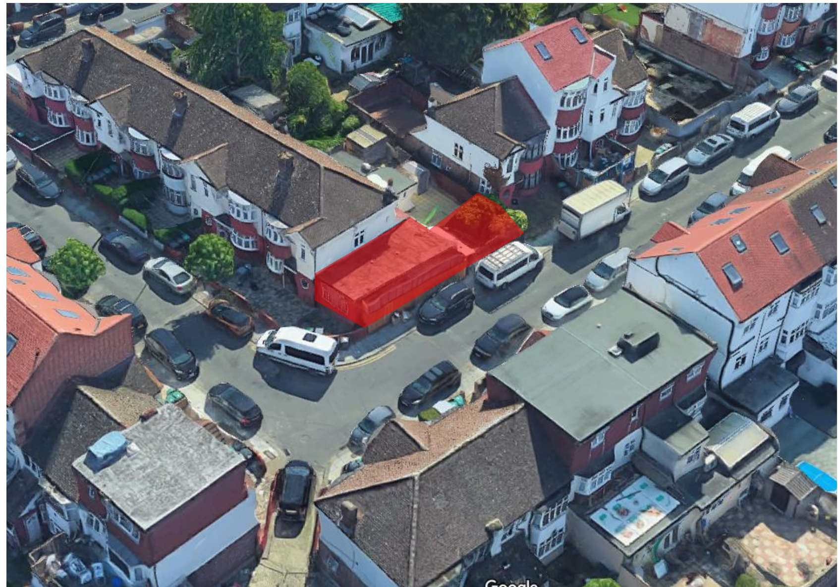
Figure 0.1 View of the Existing site
