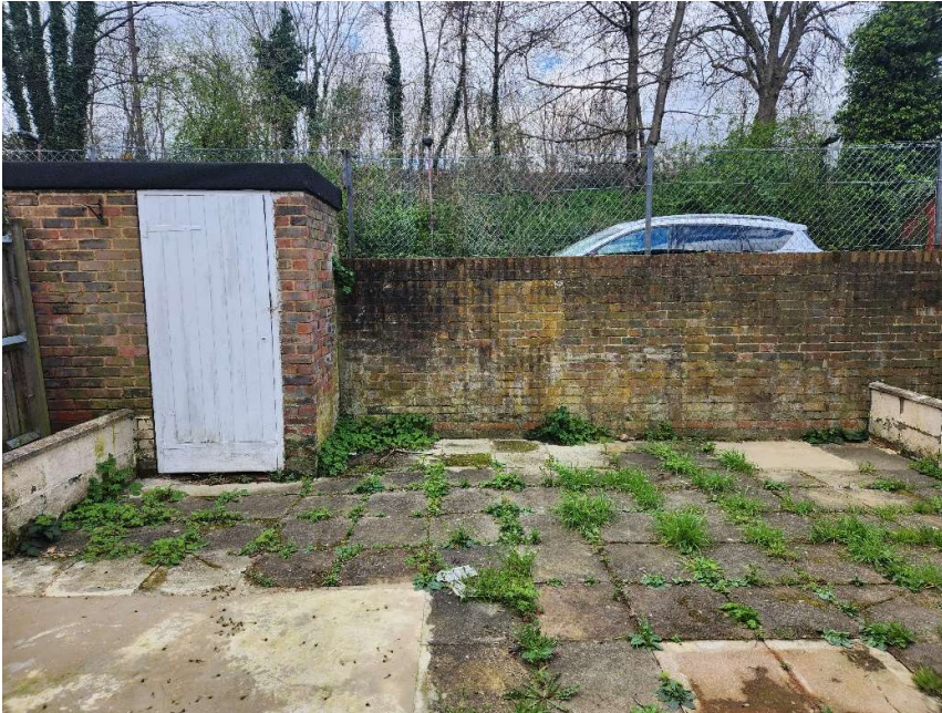
Pic 3 – View to rear boundary
