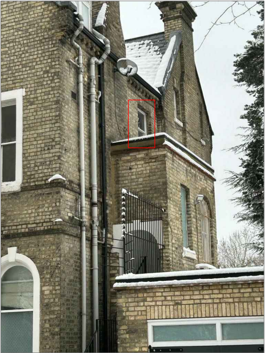
Photo of existing
