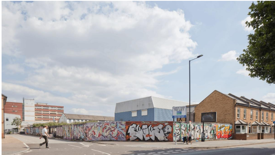
EXISTING SITE VIEWED FROM BROAD LANE
