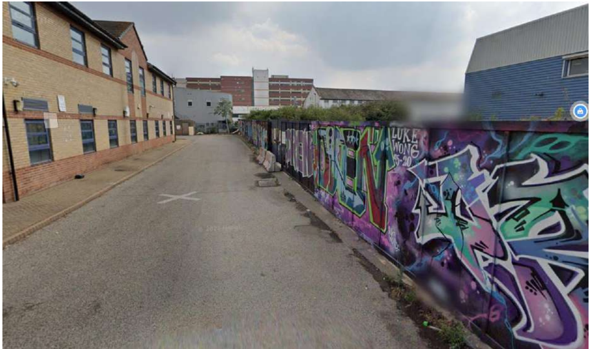
Plate 3.2: Existing site frontage
