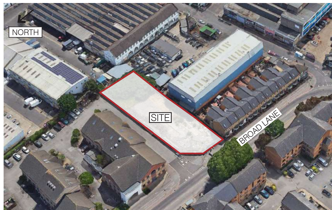
2. EXISTING AERIAL VIEW OF SITE
