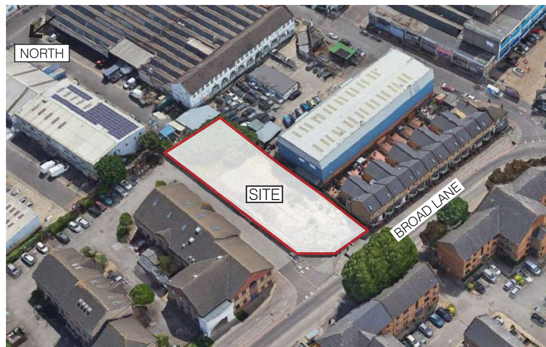
2. EXISTING AERIAL VIEW OF SITE
