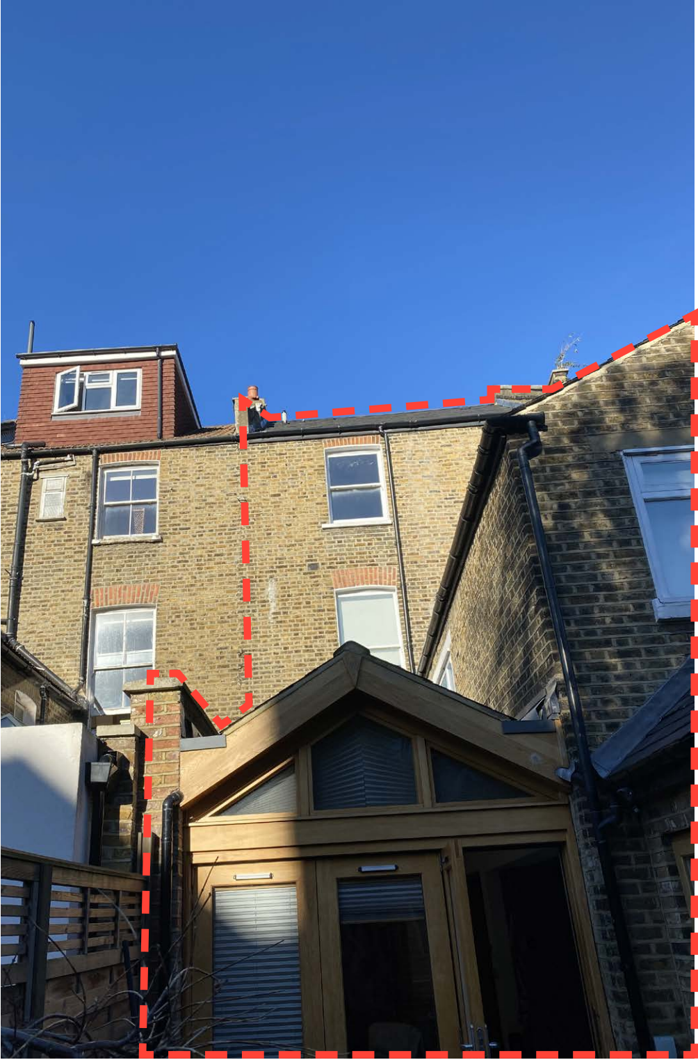
Photo of rear of building
