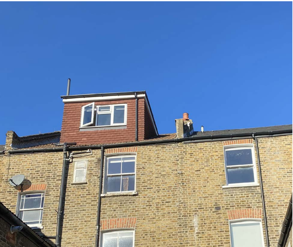
26 Stapleton Hall Road
