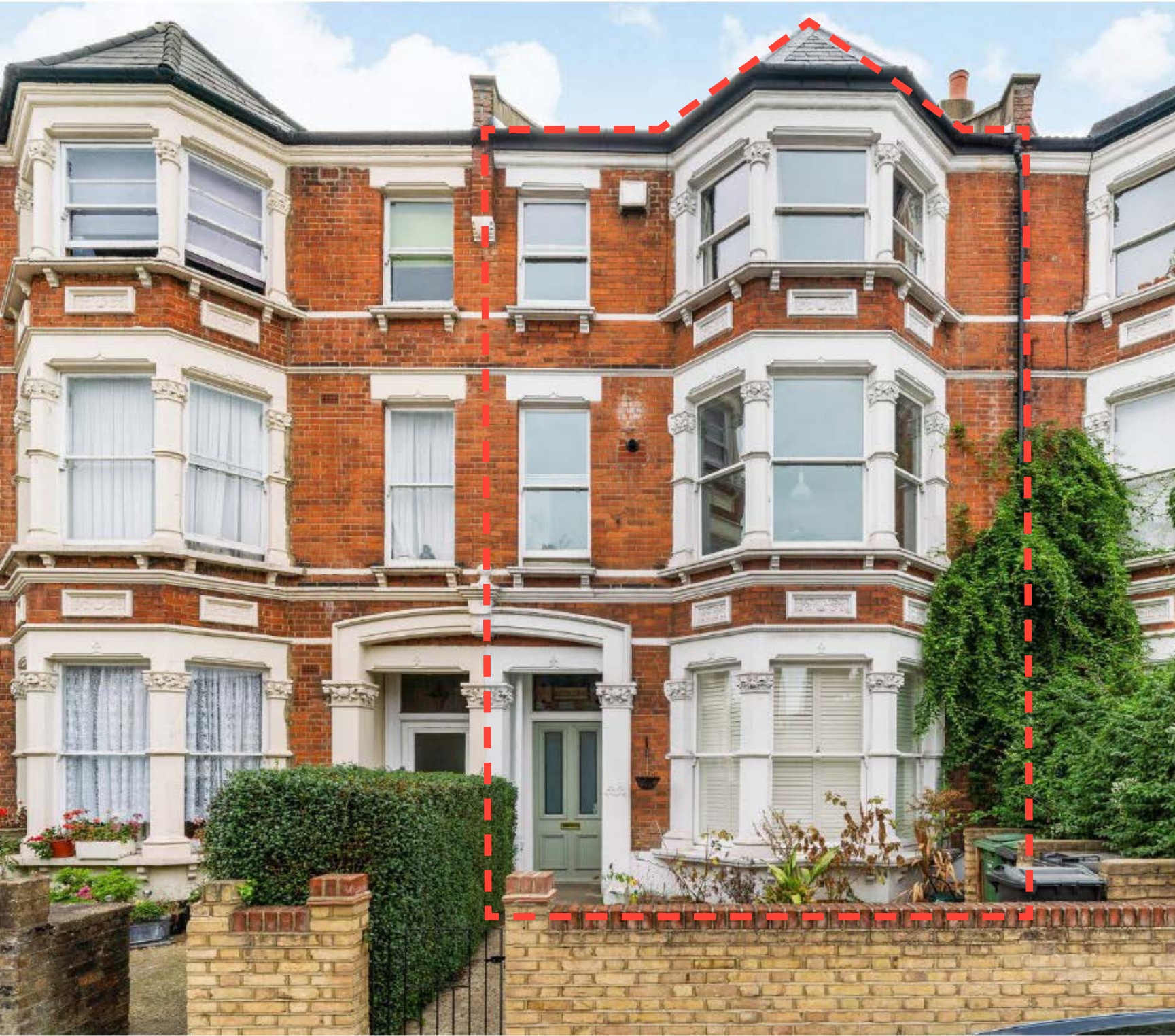
Photo of front of building
