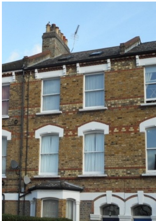
Image 4. Existing rooflights at No. 105
