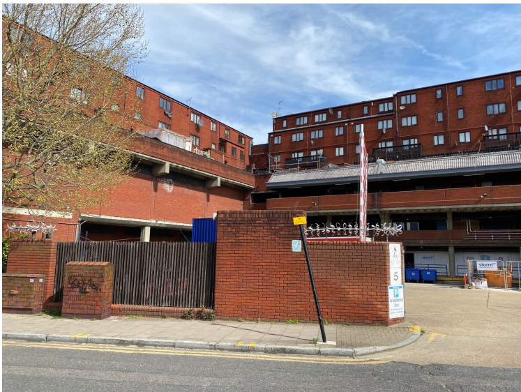
External view of site for new sub- station enclosure from Mayes Road
