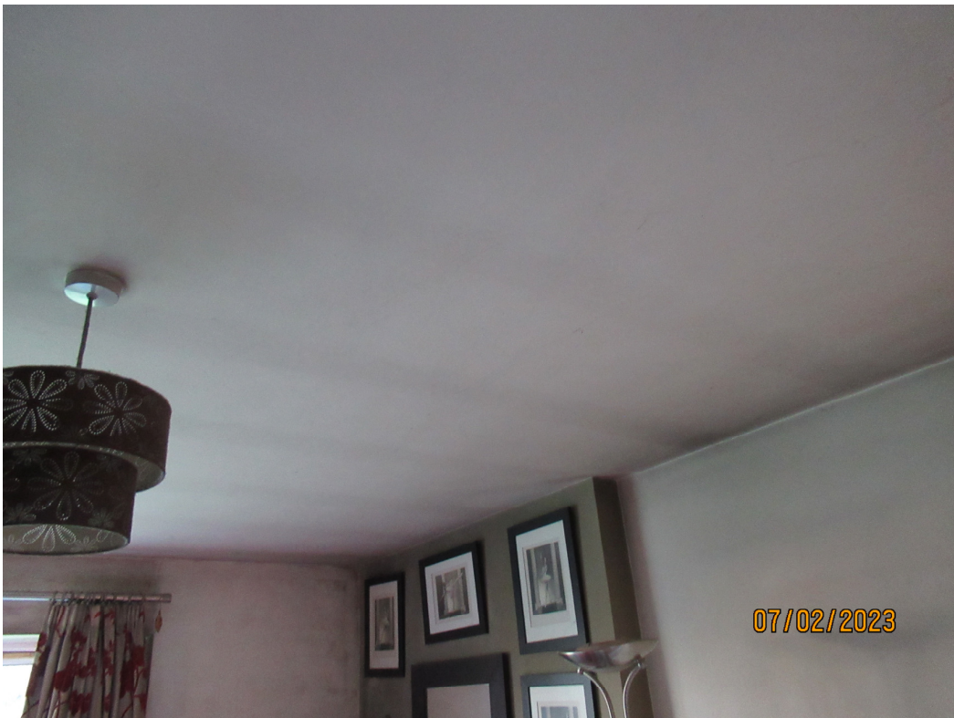
Ceiling pattern in 4, probably beam & block floor above
