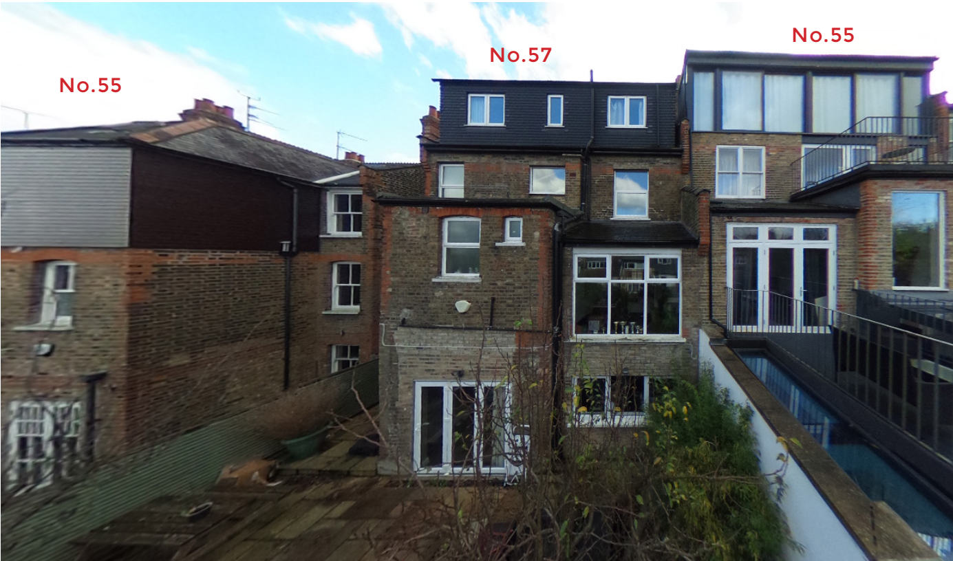
Existing rear view
