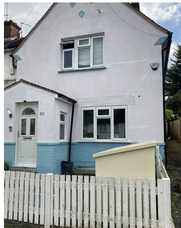
80 Barrenger Road - Metal bike storage
