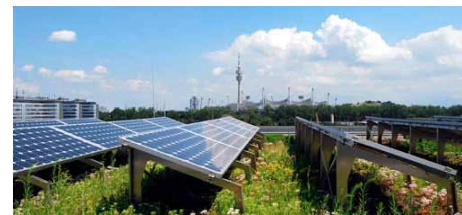
An example of a Biodiverse green roof & PV panels
