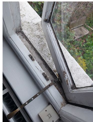
Below: Poor condition - splitting, showing signs of damp and rot caused by condensetion
