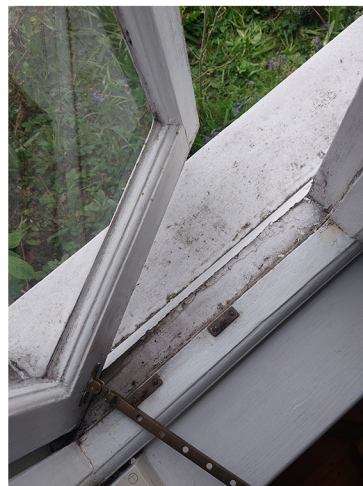
Below: Poor condition - splitting, showing signs of damp and rot caused by condensetion
