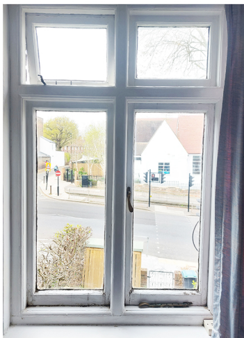
Below: Poor condition - splitting, showing signs of damp and rot caused by condensetion
