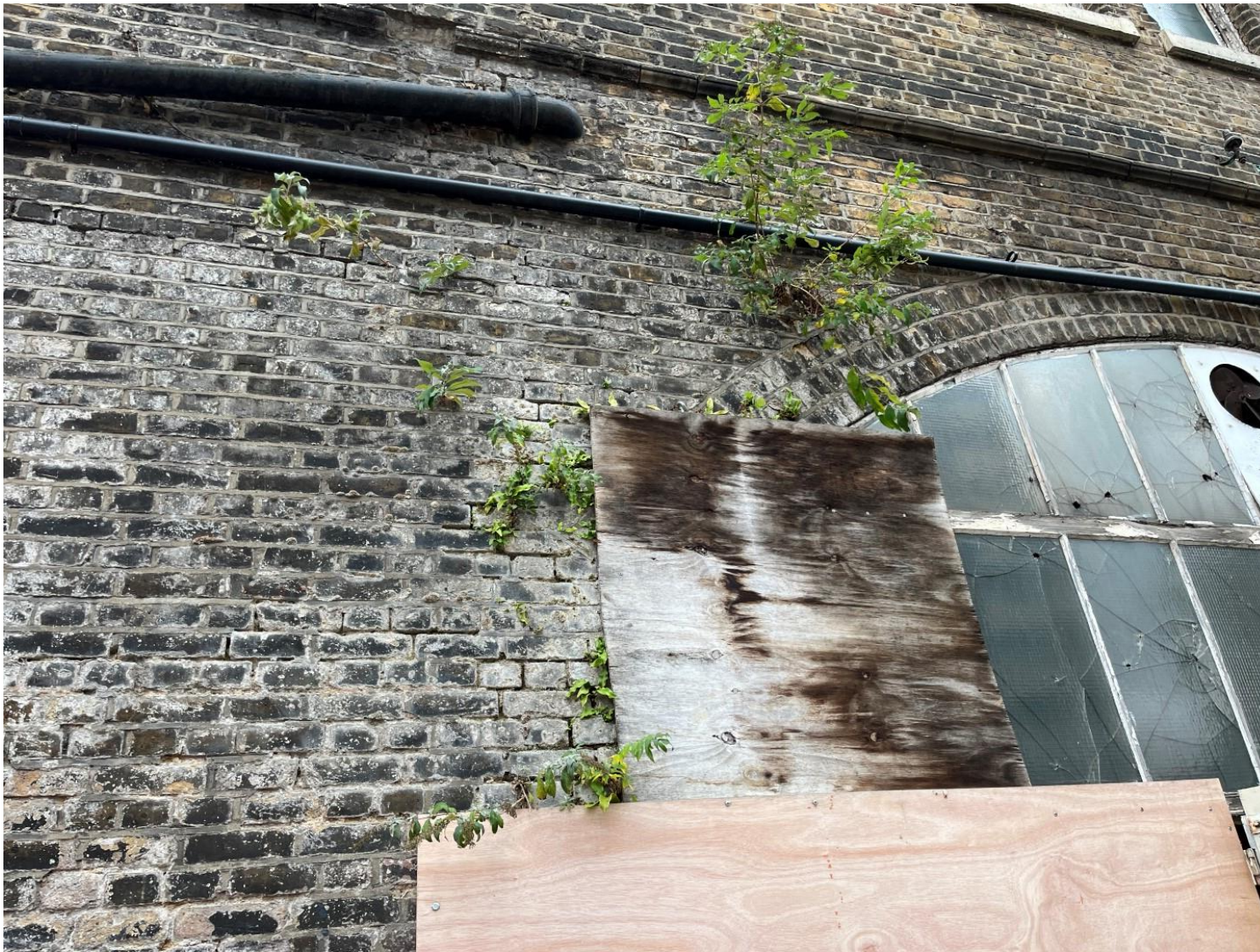
Figure 1 – Photo showing vegetation to be removed from the front elevation.
