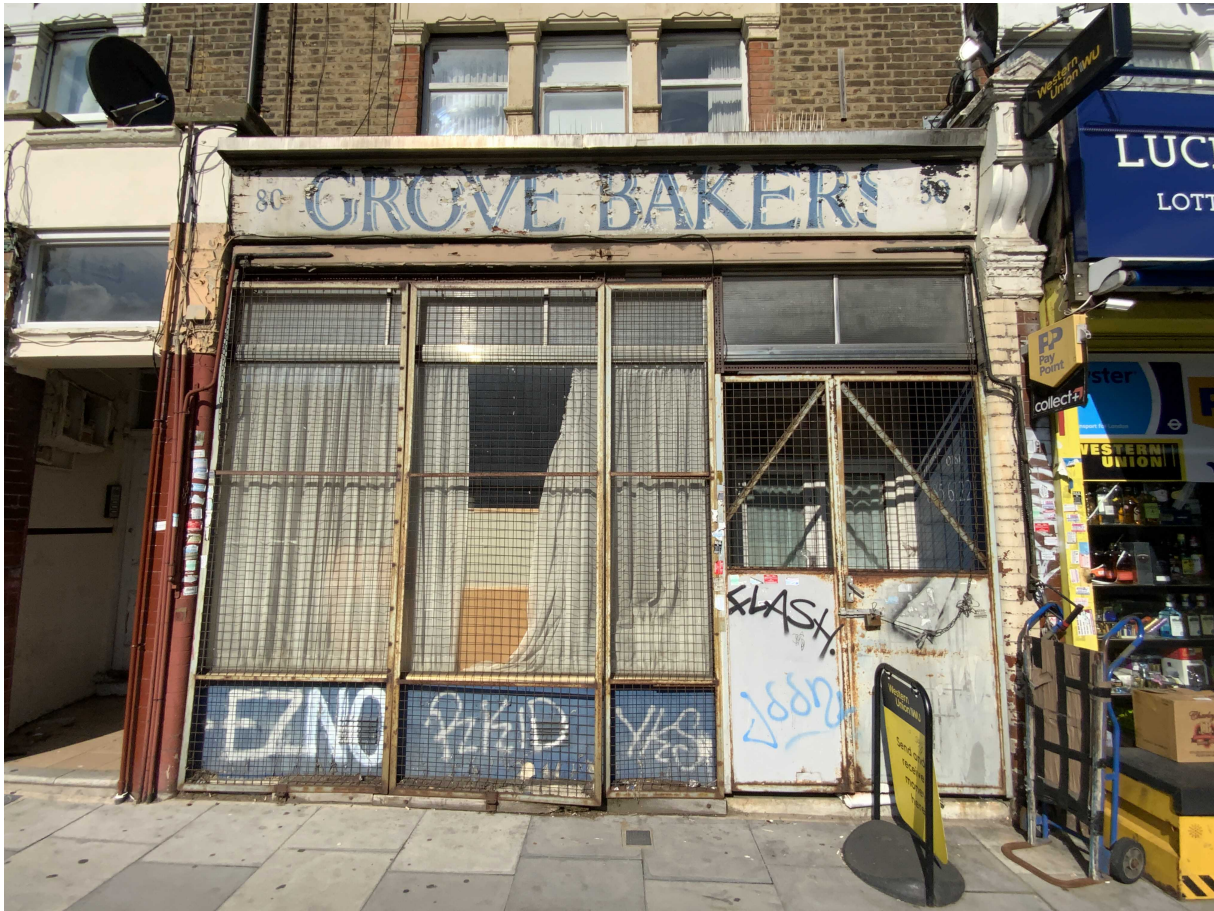
80 Bruce Grove - Shopfront - Front view
