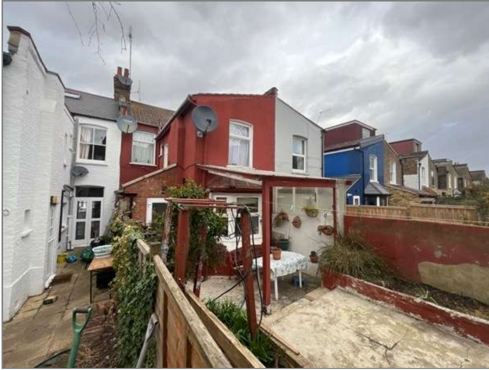
View - Rear Neighbouring Elevation
