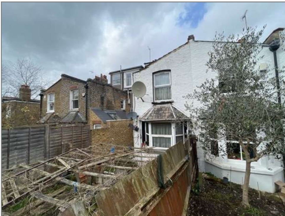
View - Rear Neighbouring Elevation
