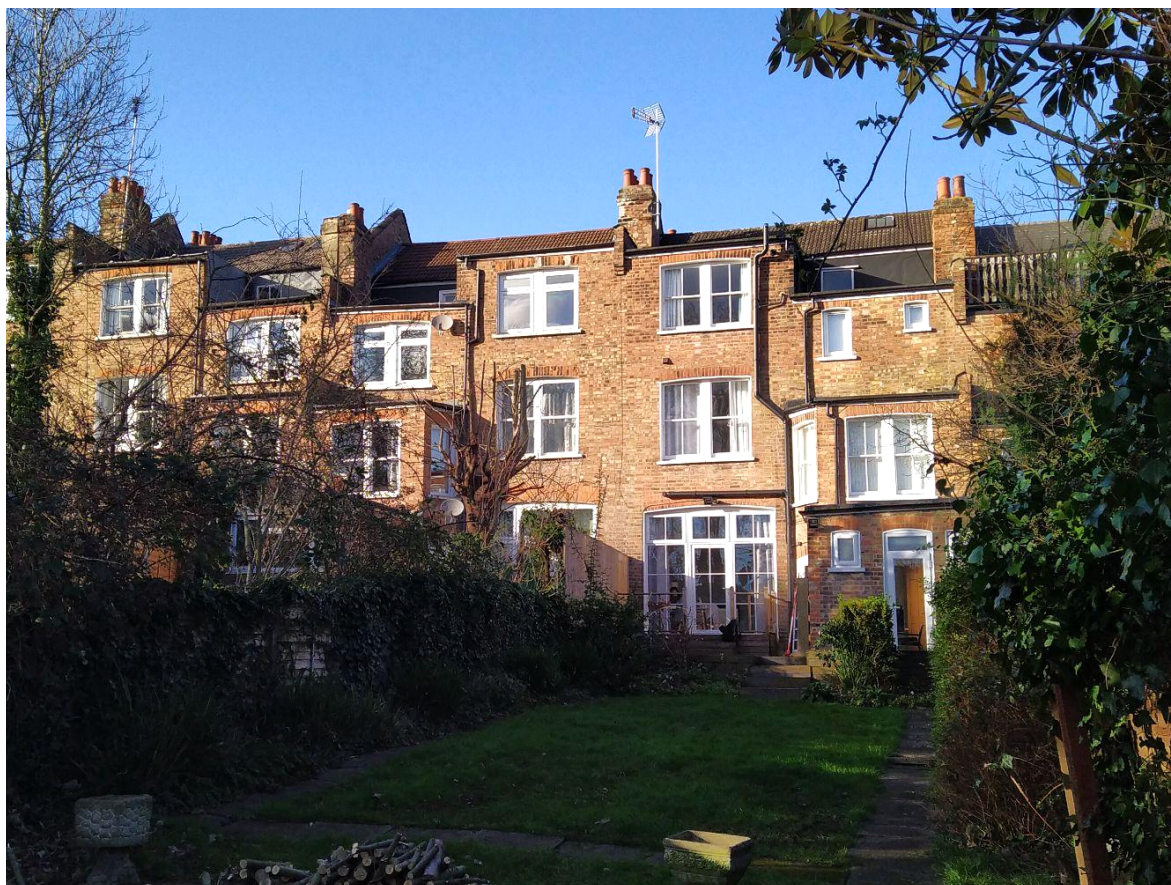
Current View of the Rear Elevation
