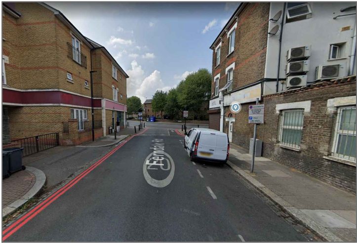
Existing Street View
