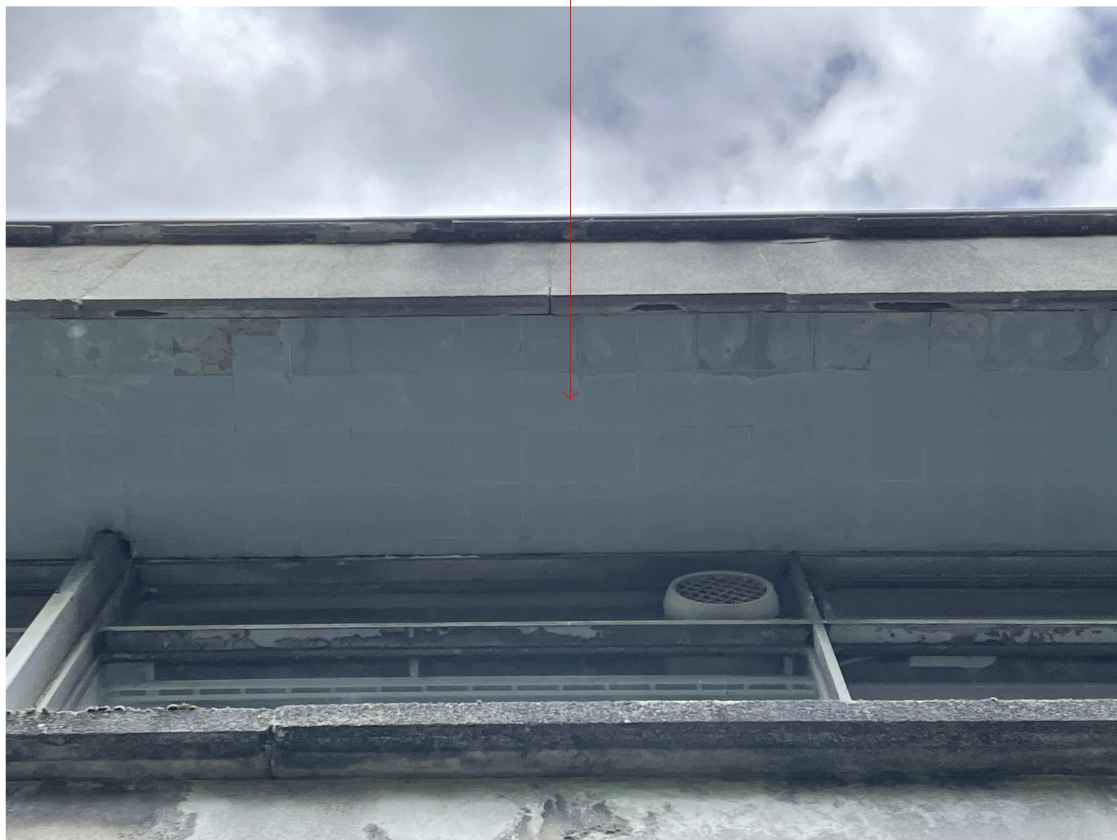
Existing condition looking up at first floor window head
