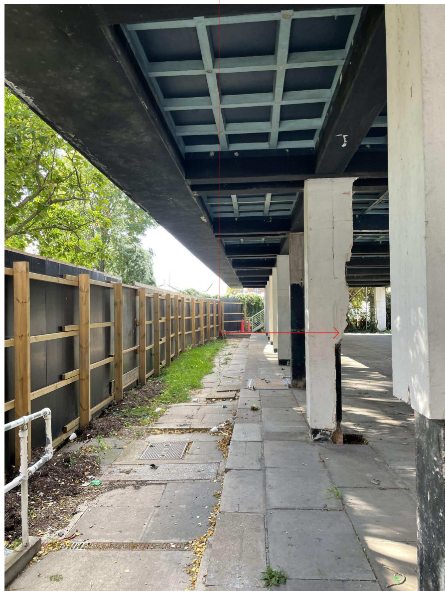
Existing condition below west wing
