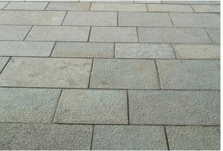
Large Concrete Paver
