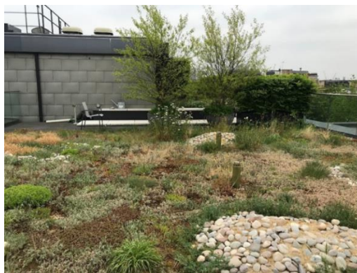
Figure 5.1 Left: Sandy piles covered in stones on biodiverse roof Right: Ephemeral wetlands on a biodiverse roof.
