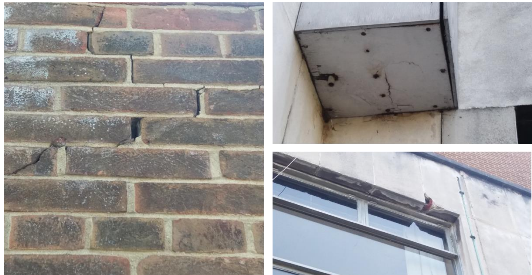
Figure 2.1 Example of roosting features on building 1.
